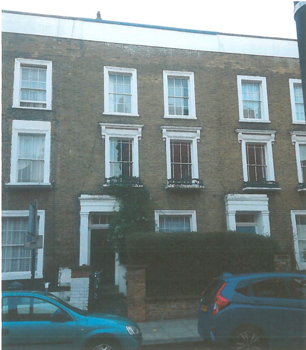
Photograph 1 - Front Elevation of 7a Grafton Road
