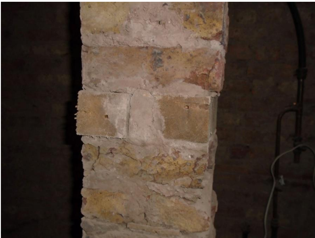
Image 15: Timber blocking embedded in brick pier approximately at mid-height
