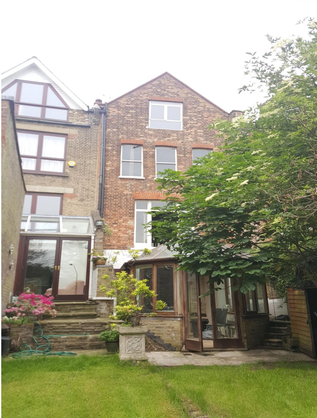
Image 4: View of rear elevation and rear conservatory
