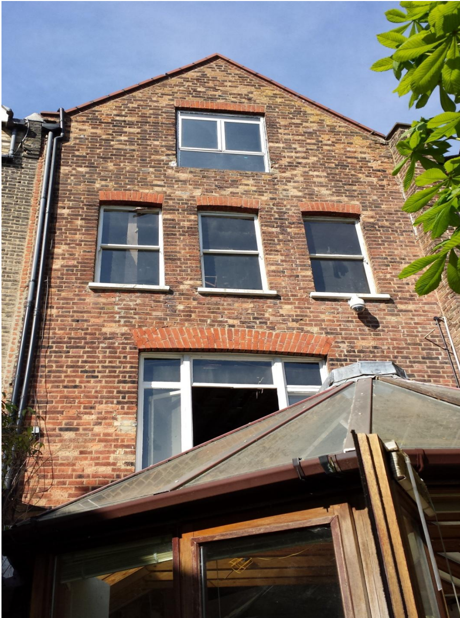
Image 3: General view of rear elevation
