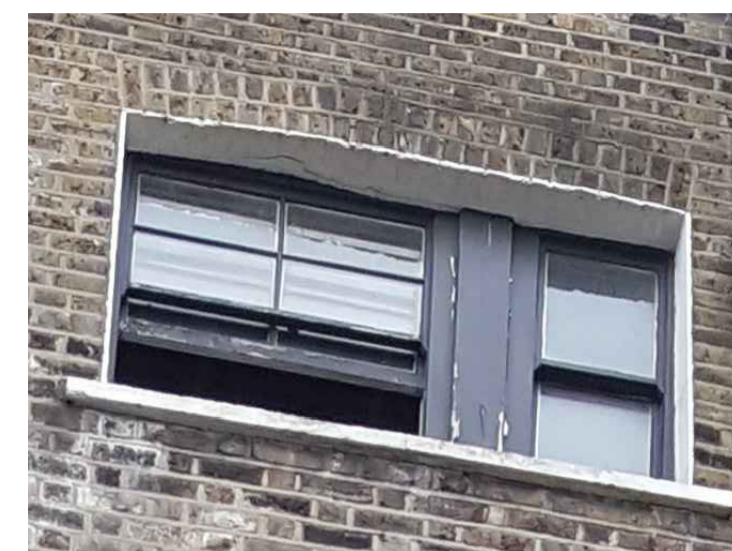
PHOTO 1 No 66 3rd Fl Rear Left Window Window No: WX.3.05
