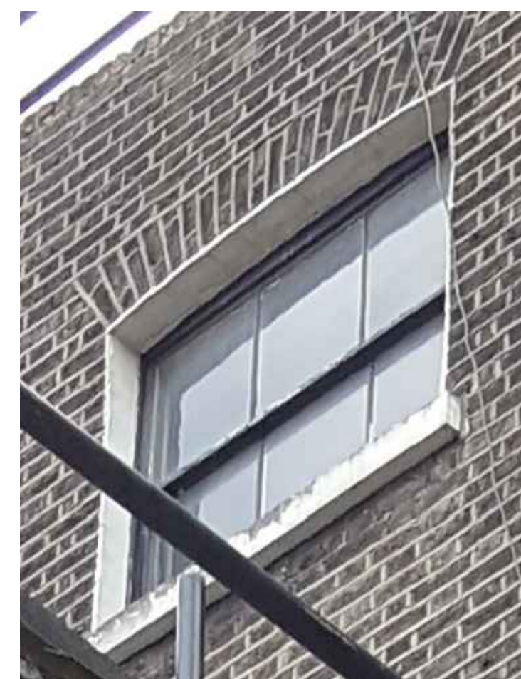
PHOTO 3 No 67 3rd Fl Rear Left Window Window No: WX.3.24
