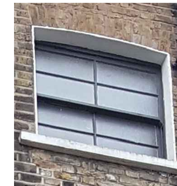
PHOTO 2 No 66 3rd Fl Rear Right Window Window No: WX.3.05
