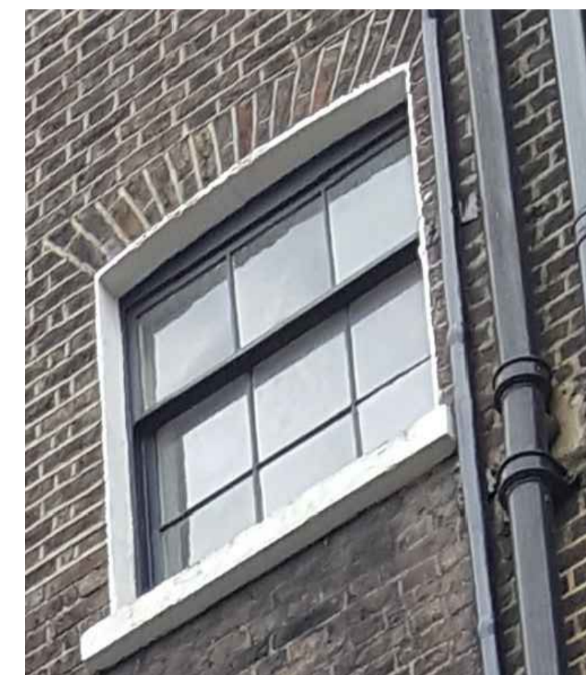
PHOTO 4 No 67 3rd Fl Rear Right Window Window No: WX.3.23
