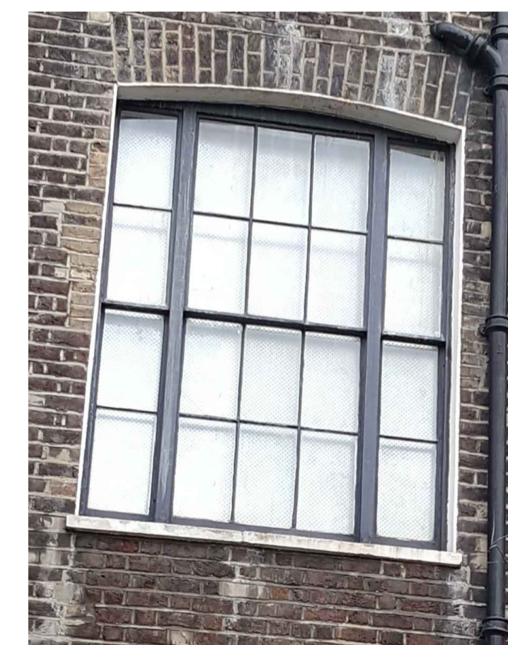
PHOTO 4 No 66 1st FI rear window Window No: WX.1.05
