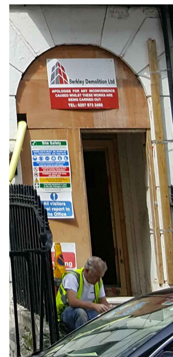
PHOTO 2 No 67 Main entrance door Door No: DX.G.20
