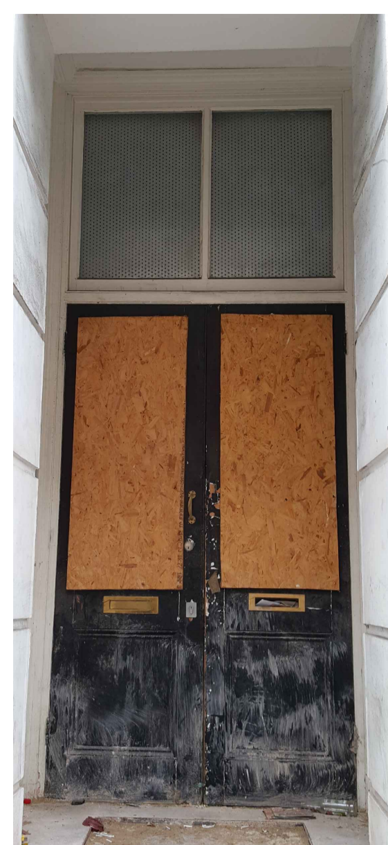
PHOTO 1 No 66 Main entrance door Door No: DX.G.01
