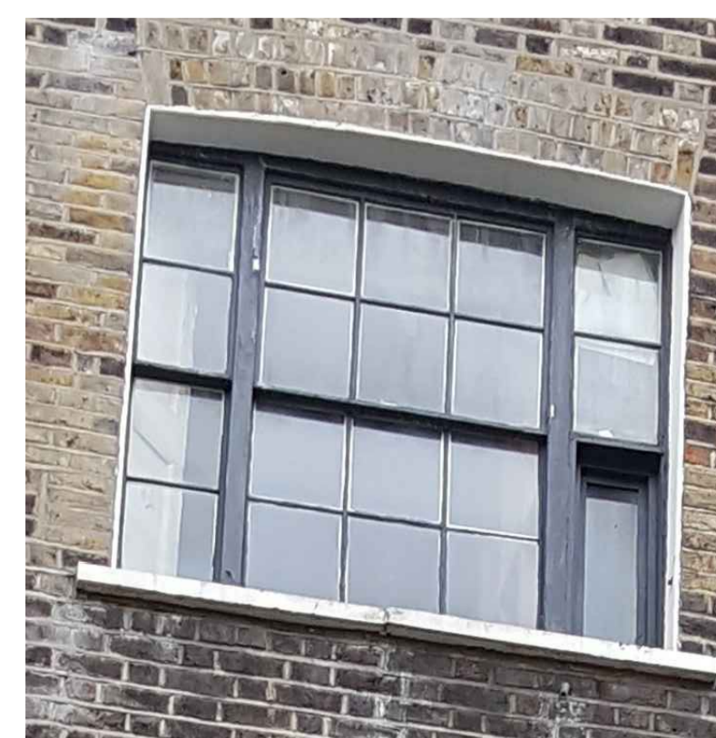
PHOTO 6 No 66 2nd FI Rear window Window No: WX.2.05
