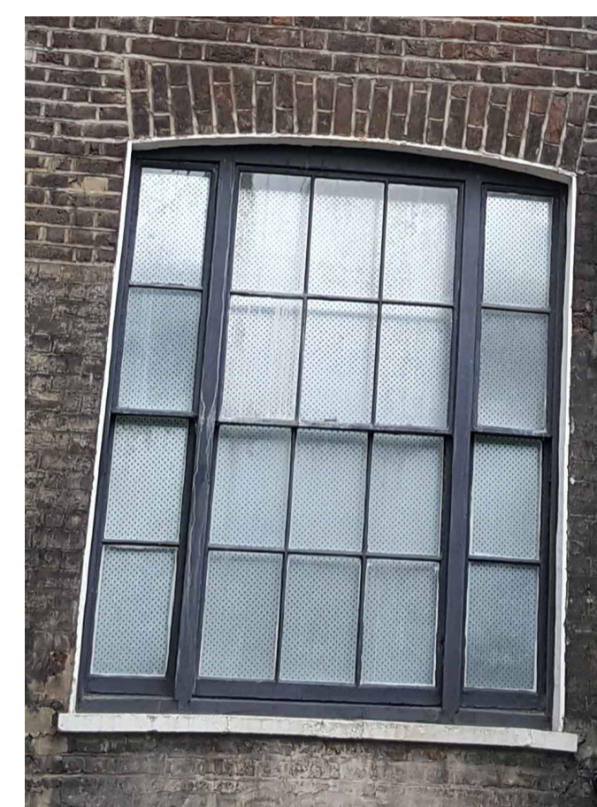
PHOTO 3 No 66 GF rear window Window No: WX.G.03
