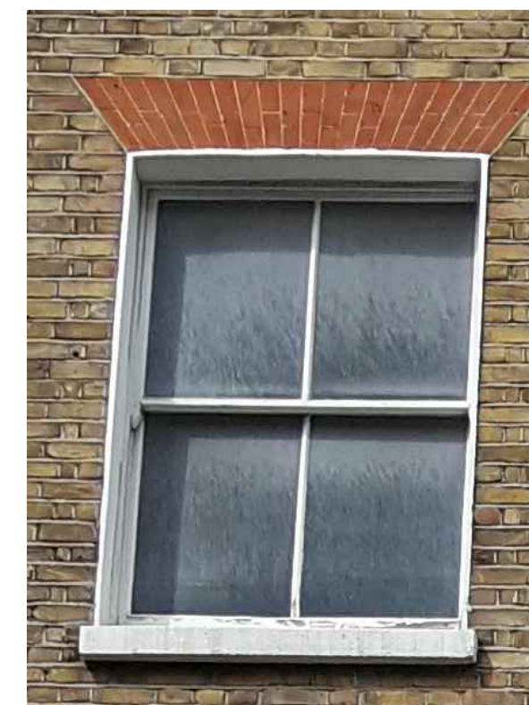
PHOTO 3 No 66 2nd Floor front windows Window No: WX.2.01, WX.2.02, WX.2.03
