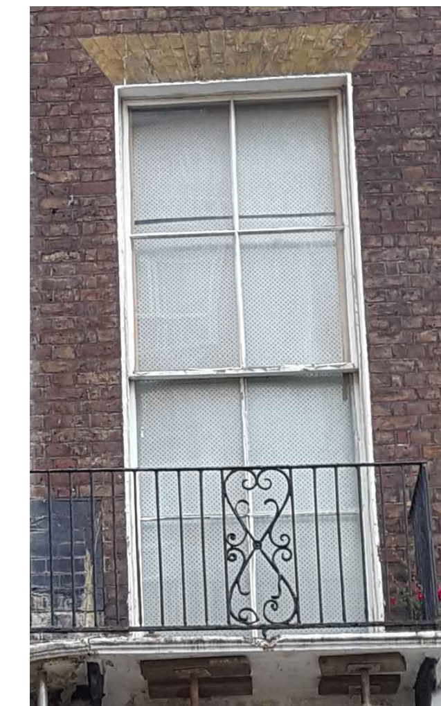
PHOTO 2 No 67 1st Floor Front Windows Window No: WX.1.20, WX.1.21, WX.1.22
