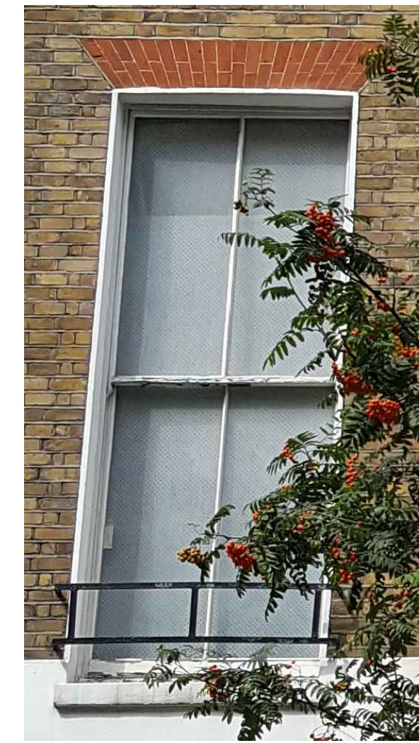
PHOTO 1 No 66 1st Floor Front Windows Window No: WX.1.01, WX.1.02, WX.1.03
