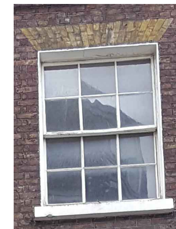
PHOTO 4 No 67 2nd Floor front windows Window No: WX.2.20, WX.2.21, WX.2.22
