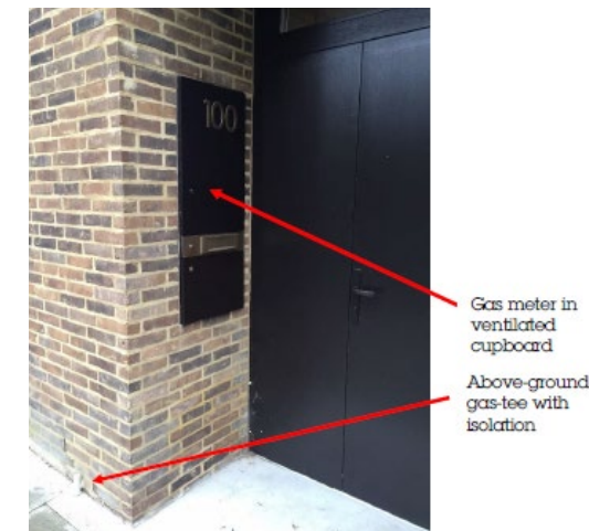
Services intakes integration within front door recess
