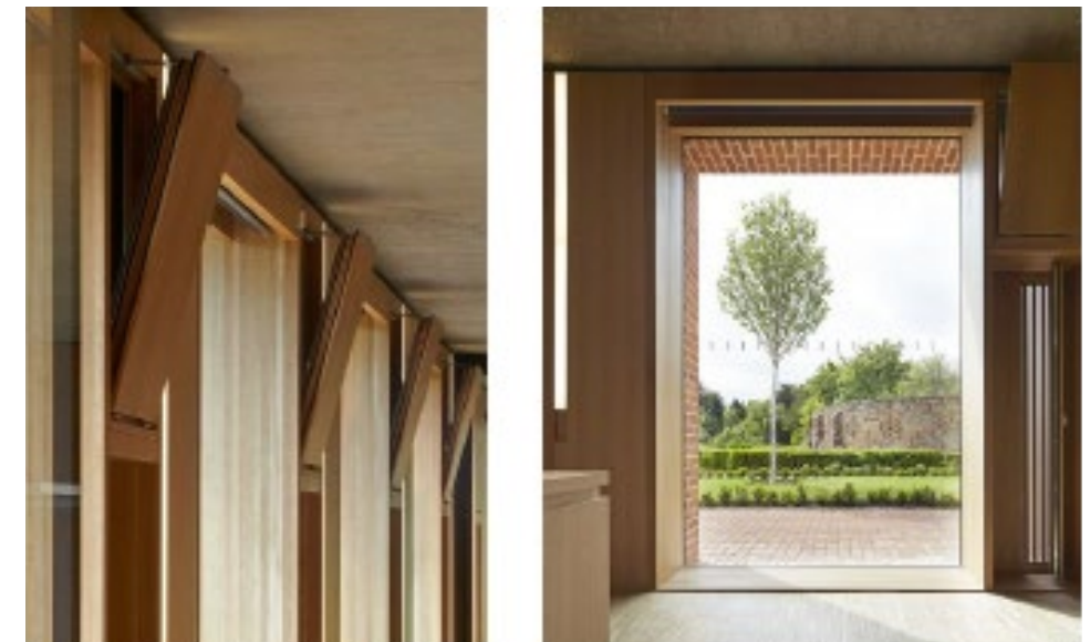
Background and purge ventilation panels
