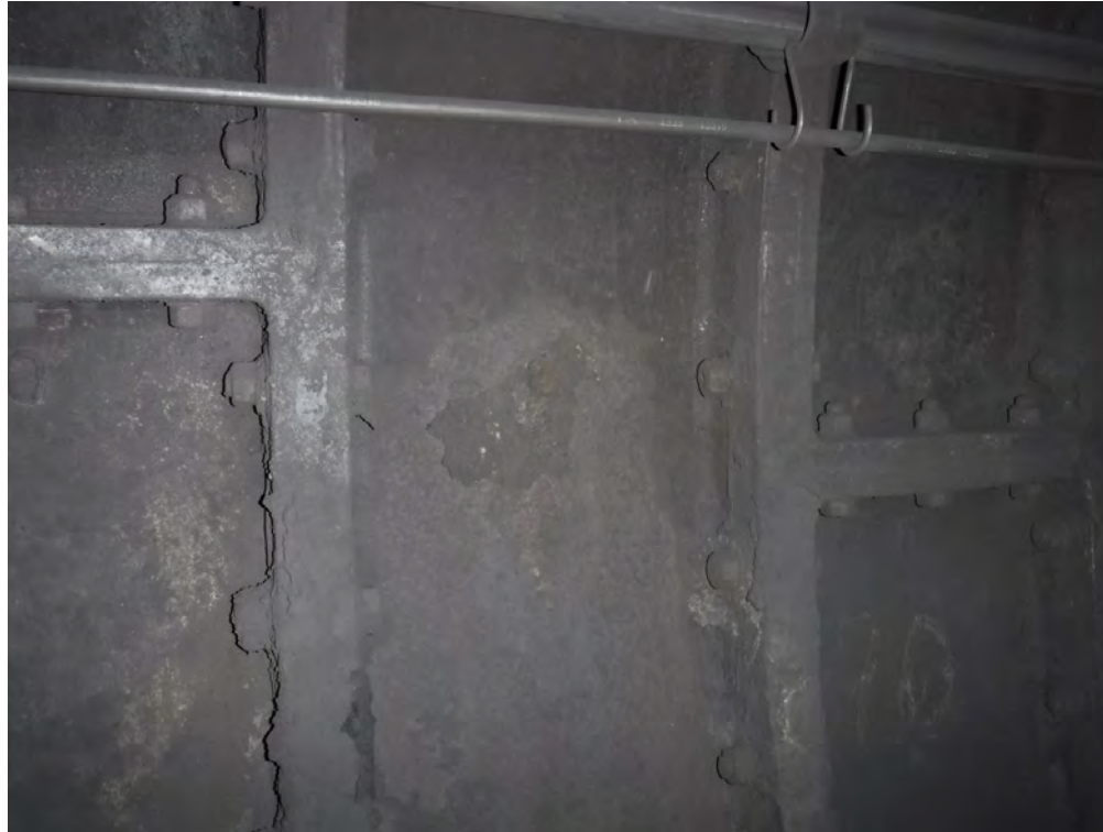
Photo-128, 40/2 @ 8 o'clock Encrustation at lifting hole of steel plate
