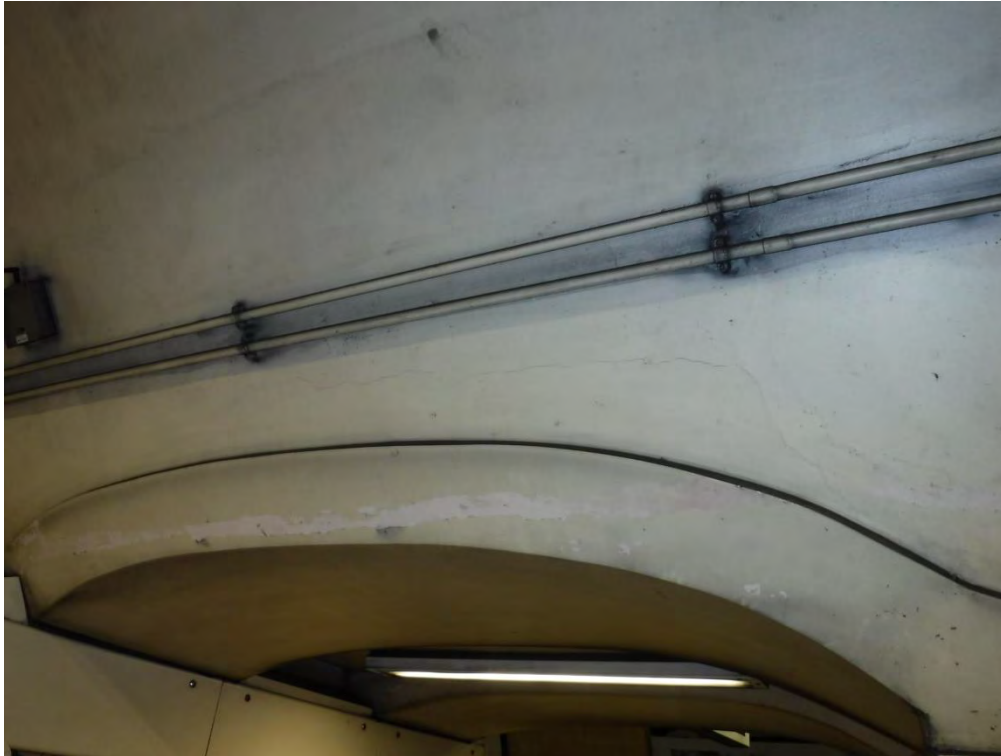
Photo-246, 1st arch to south bound tunnel Horizontal crack in render over length of arch
