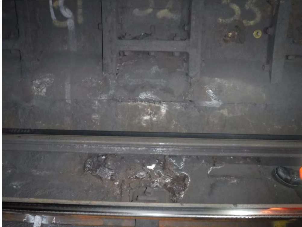
Photo-196, 20/4 @ 5 o'clock Encrustation at lifting hole of steel plate
