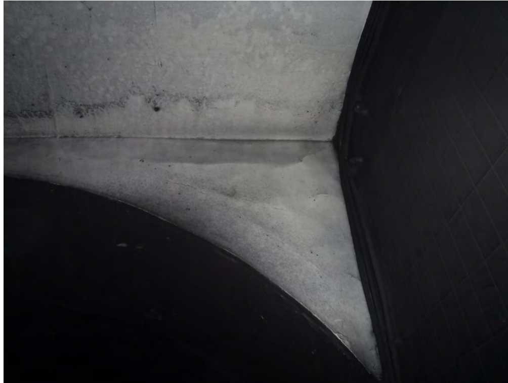
Photo-238, South end head wall @ 11 o'clock cracks in render of head wall
