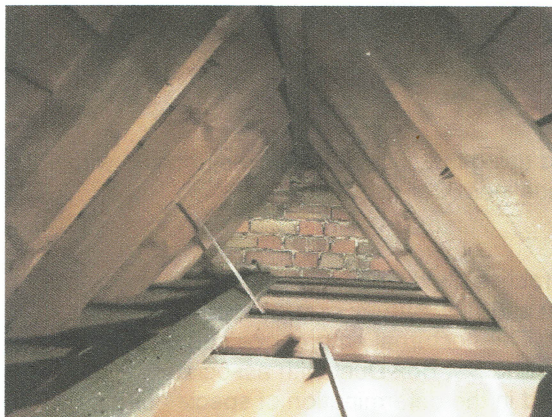
Plate 1: Small Roof Void Left After Loft Conversion
