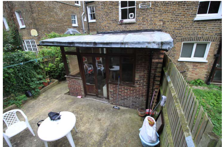
Existing rear extension
