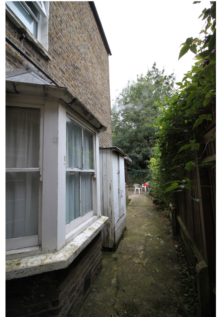
Side passage looking west
