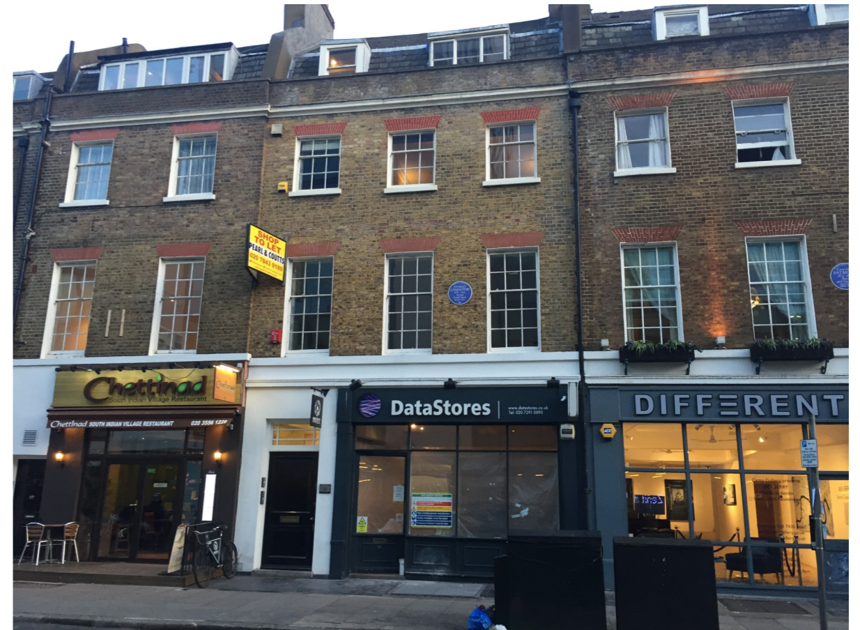
Plate 1: Front Elevation of No.15 Percy Street
