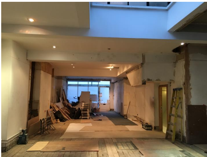
View of Interior looking towards shopfront
