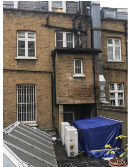
View of air-conditioning at rear
