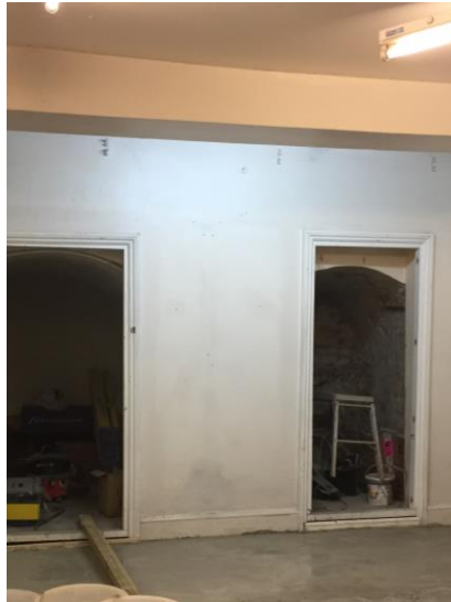
View of existing vaults at basement level
