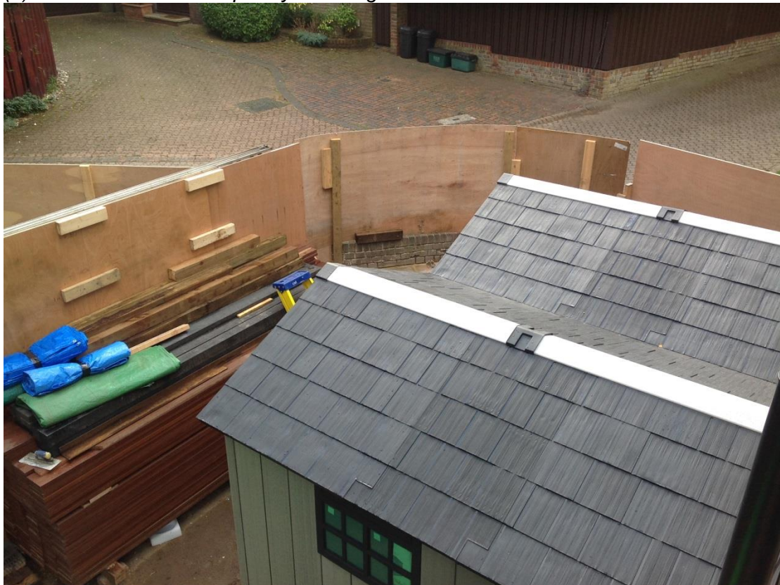
(9) Garden area with temporary hoarding and office
