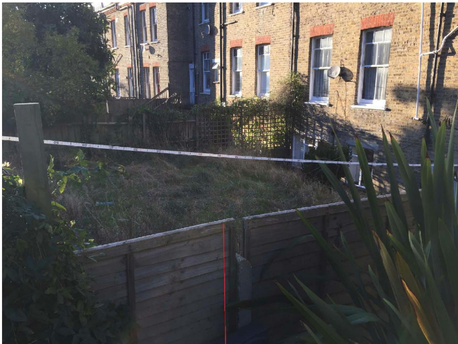
Another shot showing the approximate 7.75m reach of the extension.
