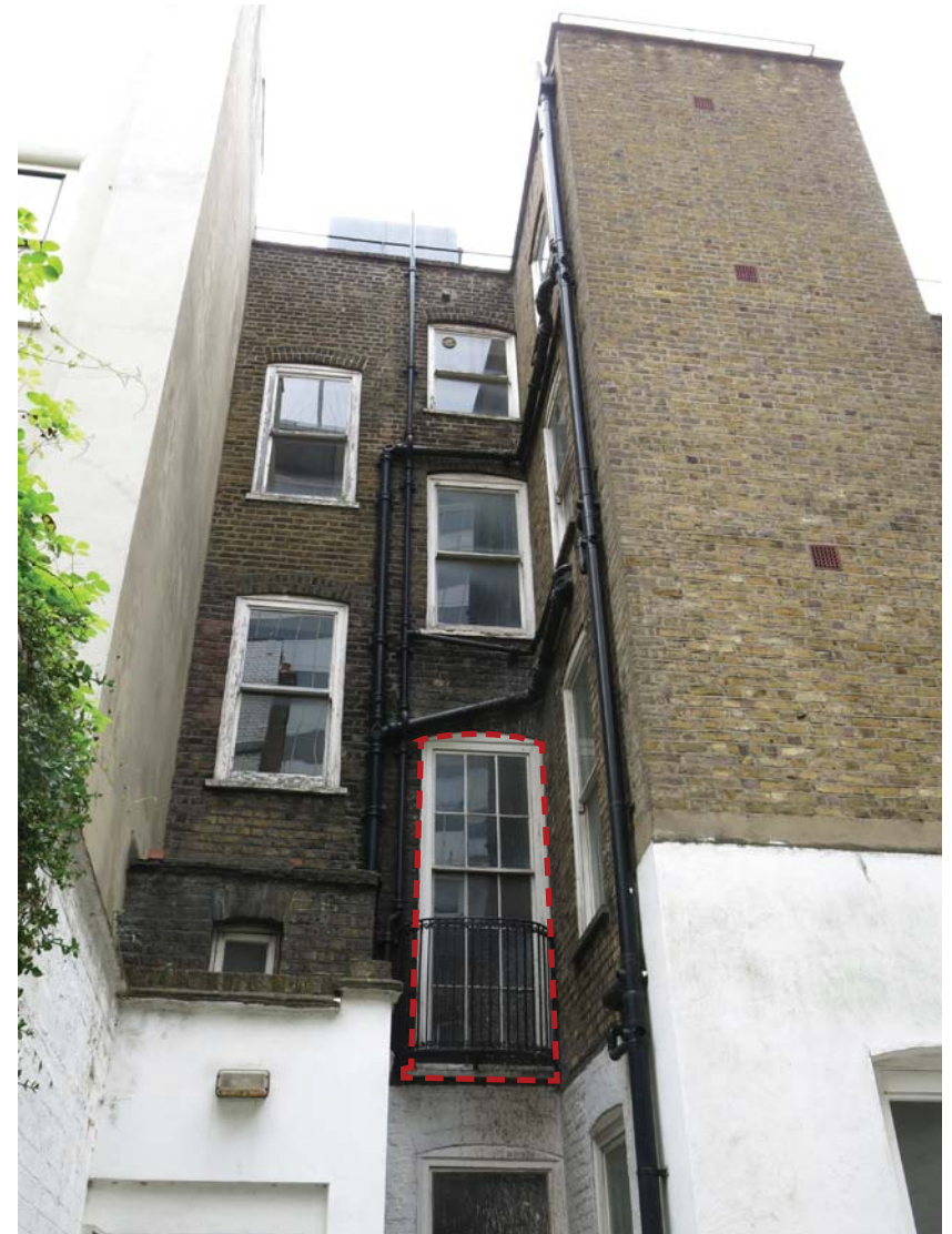
Fig.4h Window lengthened in the Regency period.
