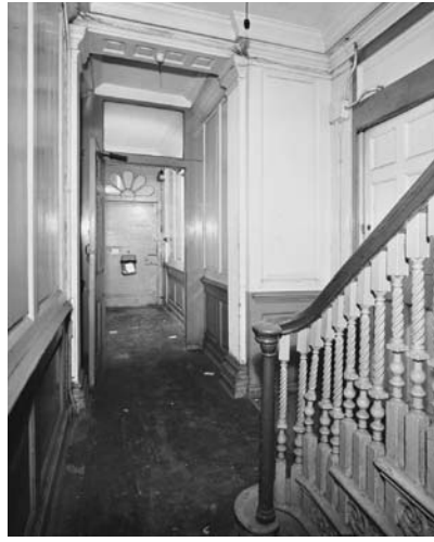
Fig.3i Photograph of entrance hall and staircase with barley twist balusters at no.31 Great James Street, 1971. London Metropolitan Archive.
