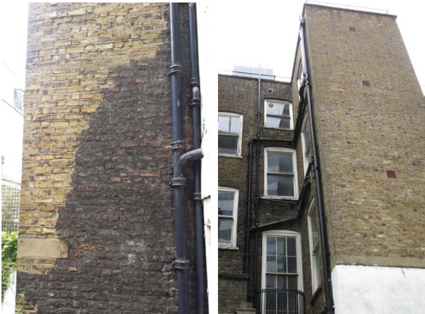
Fig.3q No. 39 - Side of closet wing, with lintel above ground floor.
