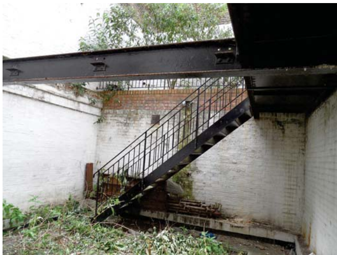
Fig.4i Bricked in backfill.
