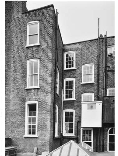
Fig.3l Photograph of rear elevation of no. 8 Great James Street showing typical WC rear extension, 1976. London Metropolitan Archive.
