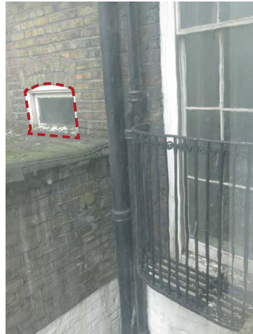
Fig.4g Window shortened to allow WC extension.
