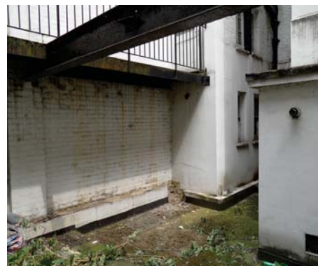
Fig.4j View showing narrow rear extension
