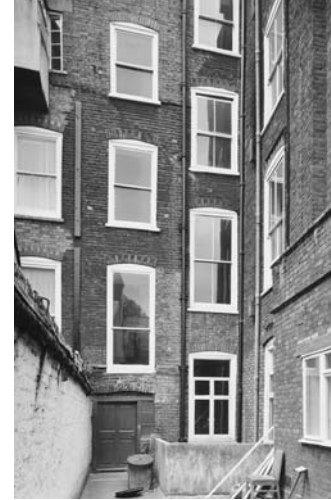
Fig.3k Photograph of rear elevation of no. 7 Great James Street showing original ground floor door and brick arch, 1971. London Metropolitan Archive.
