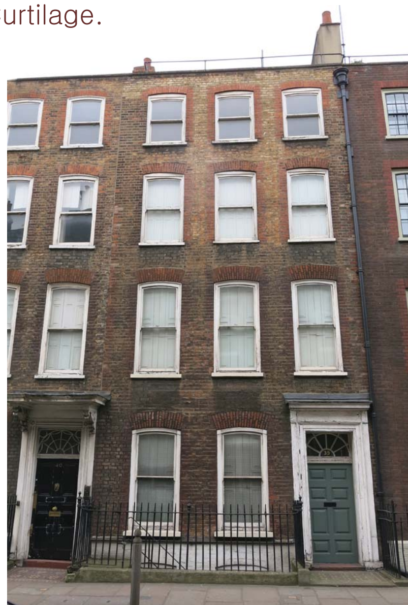
Fig.4c Front elevation of the property.
