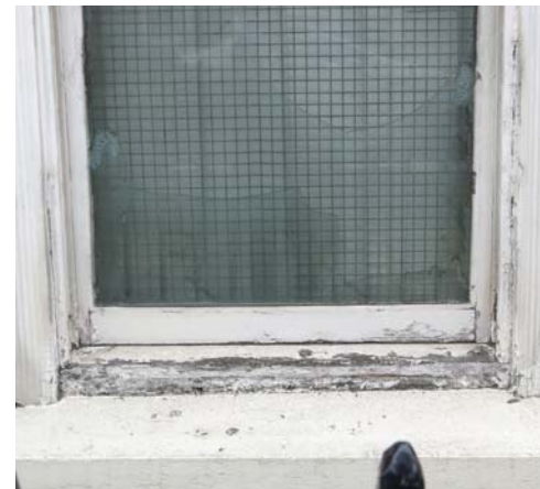
Fig.4e Ground floor windows on front elevation.
