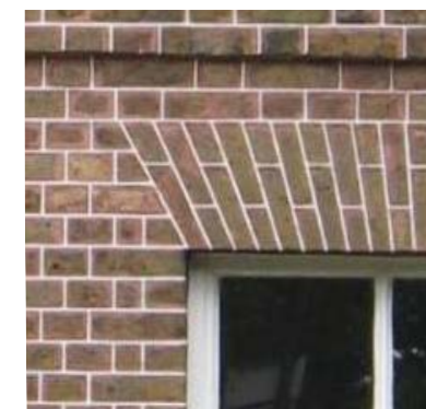
Fig 3b. Example of tuck pointing.
