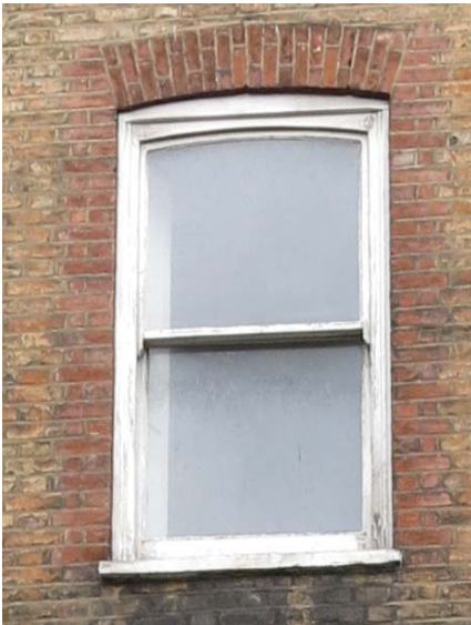
Fig 3v. Photograph of existing sash windows without glazing bars.
