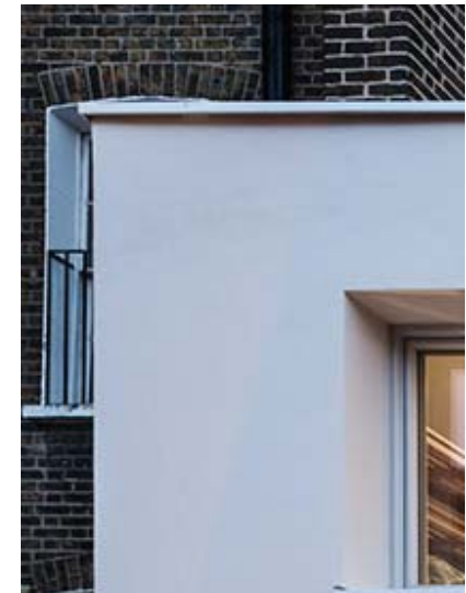
Fig 3iv. Photograph of off white painted lime render at John Street, Bloomsbury.
