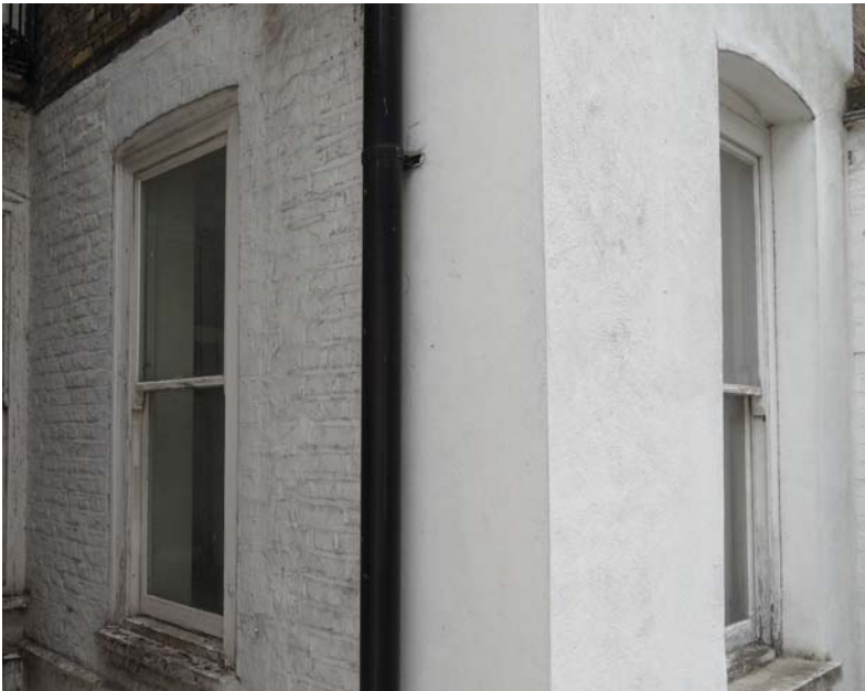
Fig 3xiv. 39 Great James Street Existing painted brickwork and render to rear of property
