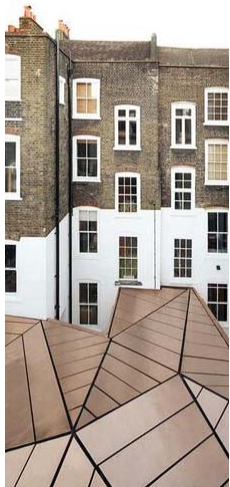
Fig 3ix. Copper roof to new extension at 32-33 Great James Street.
