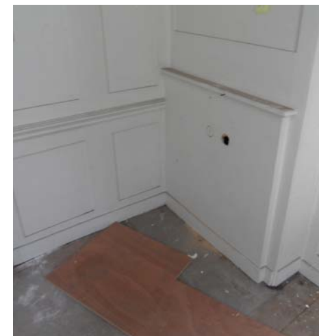
Fig 3i. 39 Great James Street: Boarded over chimney piece, ground floor closet wing.
