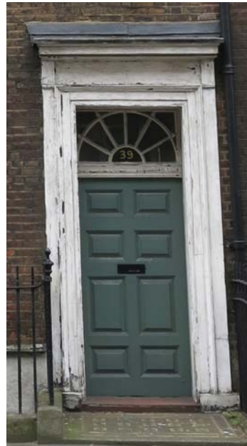
Fig 3xv. 39 Great James Street Existing front door
