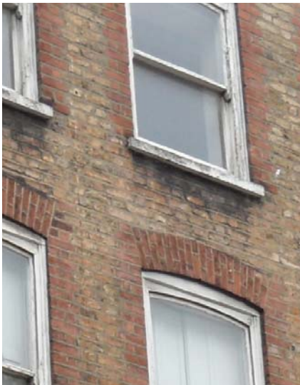
Fig 3i. Existing brickwork to front elevation of property.
