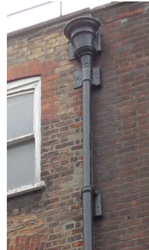
Fig 3xii. Photograph of existing metal rainwater hopper and downpipe.
