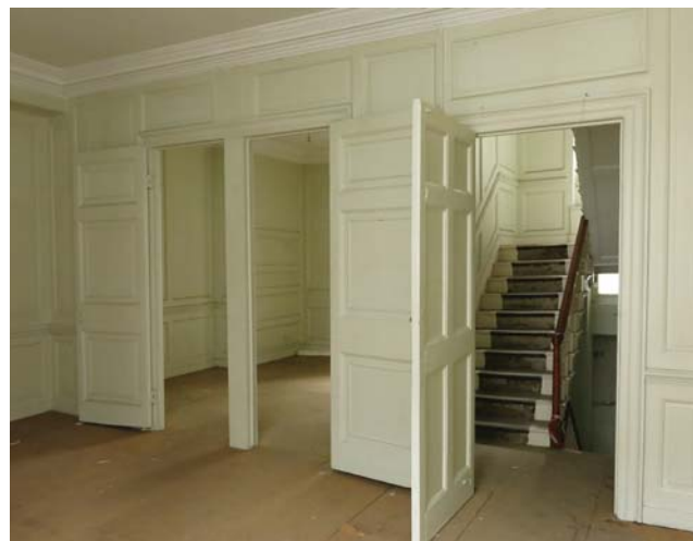
Fig 3h. 39 Great James Street. Existing interiors on First floor showing double doors from the 1970s.
