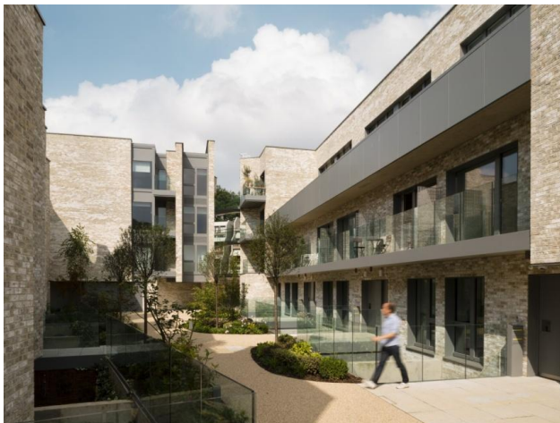
Fig.3 Existing view internal of courtyard
