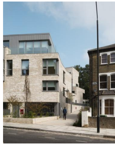
Fig.4 Existing view from Chester Road looking towards public footpath
