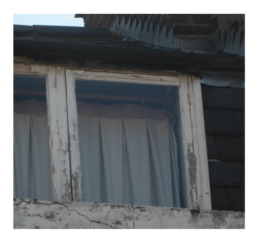
Rather than carry out extensive repairs on the existing dormer the owner prefers to replace the dormers to match no 34, the adjoining property.
