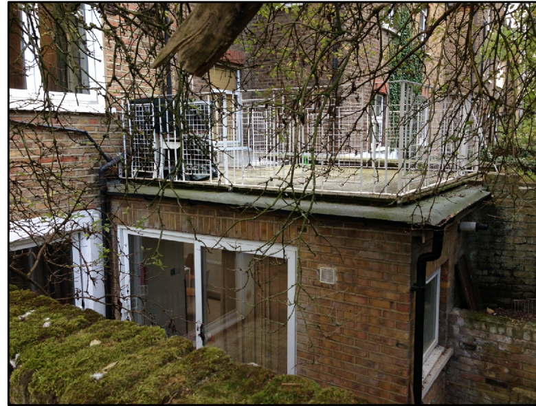
Adjacent property extension
