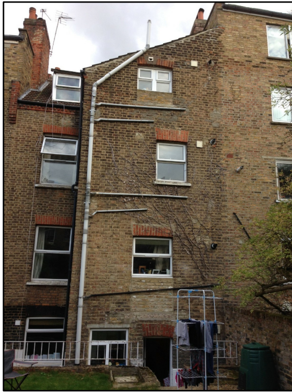
Rear of 9 Kingdon Rd
