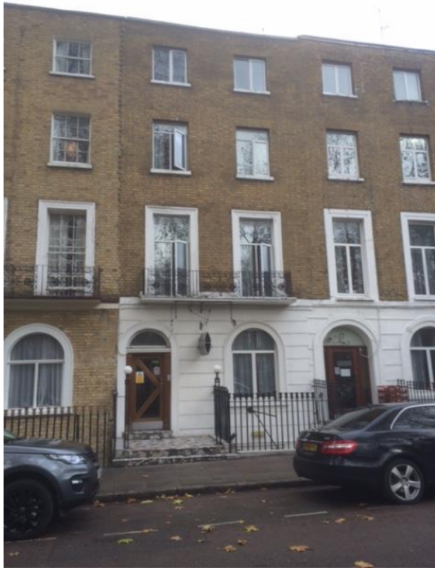
3. Pre-existing photograph of Hotel Montana, 16-18 Argyle Square (copied from planning statement)
