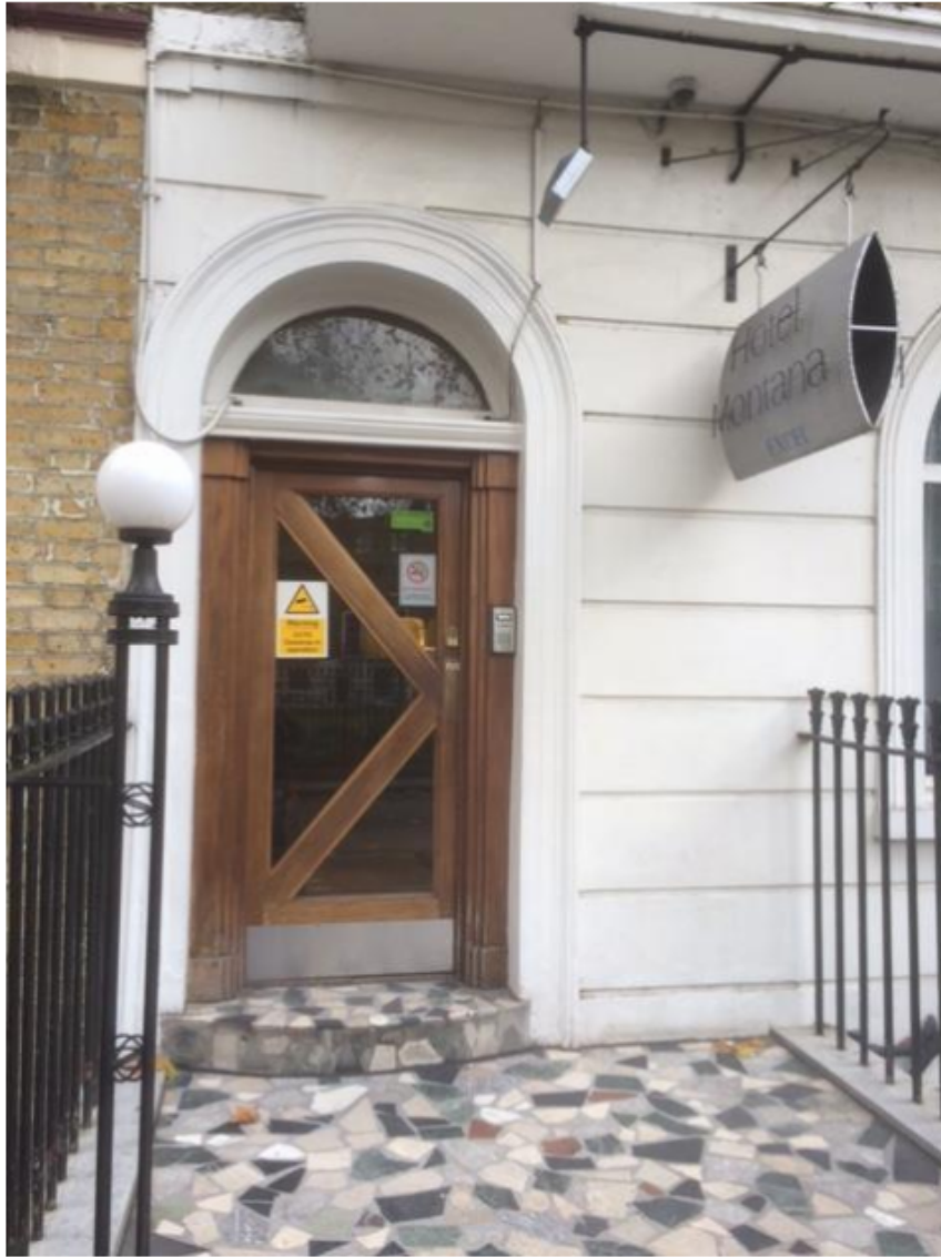
5. Photograph of existing front door of Hotel Montana (entrance to 16 Argyle Square)
