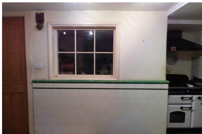
Photo 3: Wall section above white & green tiling to be removed
