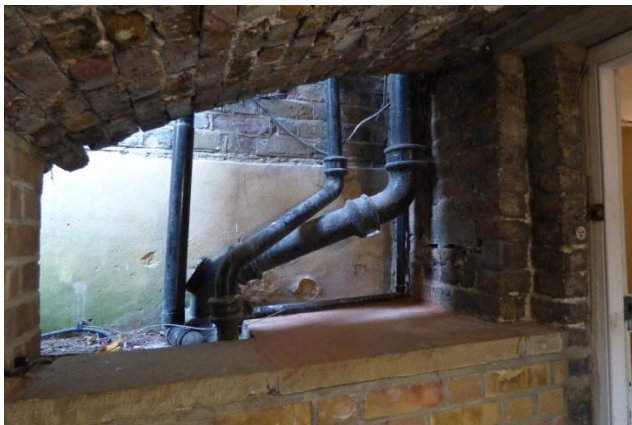
Photos 9 and 10: Downpipes passing front door to the trap within modern brick 'box'.
