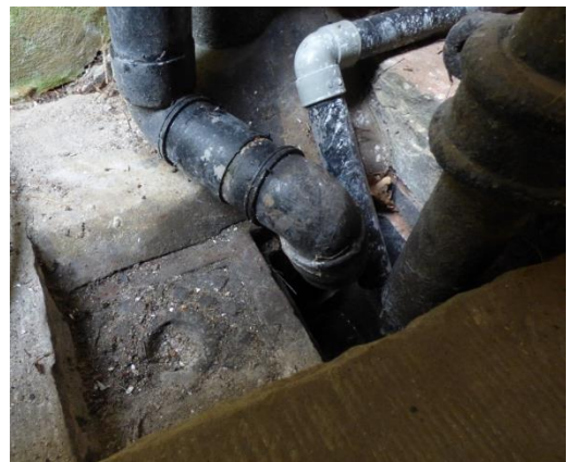
Photos 9 and 10: Downpipes passing front door to the trap within modern brick 'box'.
