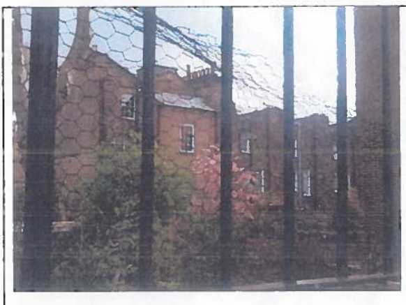
3. Rear Carol St ,adjacent property showing extent of ... Mansard roof
