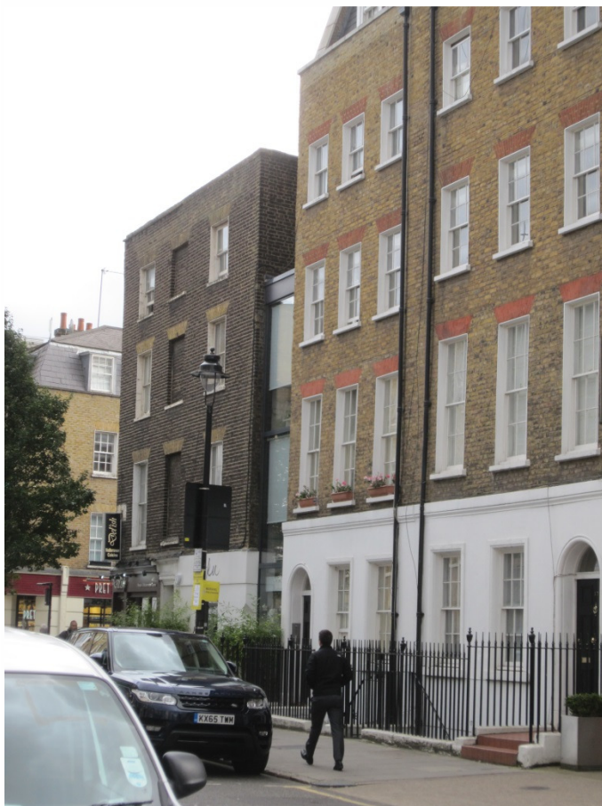
15a Warren Street from the West
