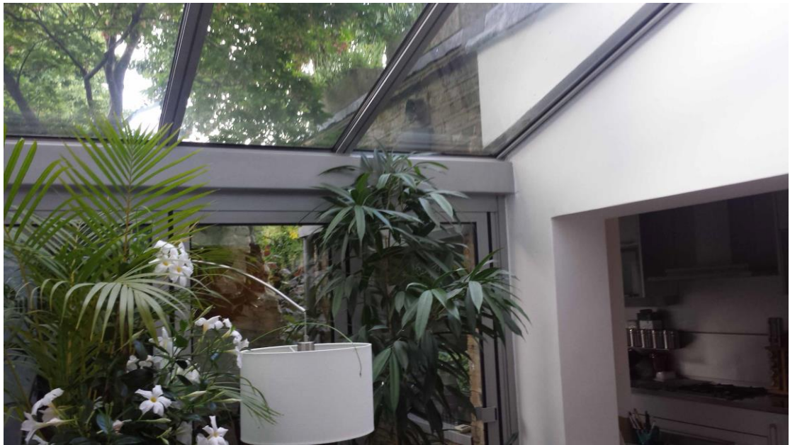
View of existing conservatory roof from inside
