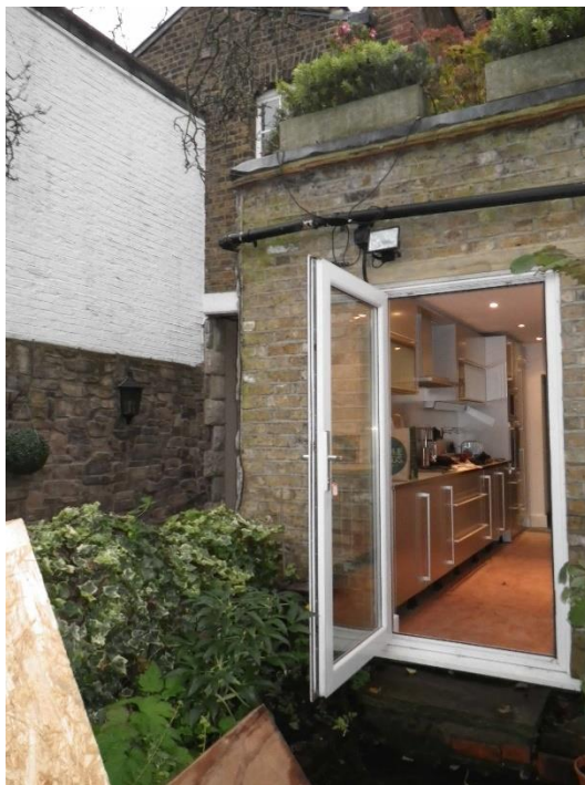
Existing rear elevation of ground floor closet wing.
