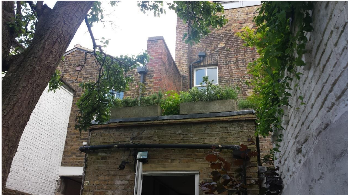
View from main rear garden looking back to existing ground floor closet wing with rear building line of adjoining lower terrace to SW boundary
