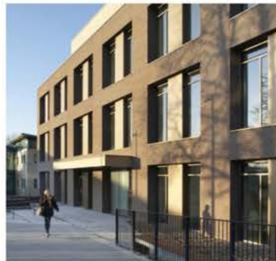
Precedent: Hawkins/Brown - Kingston Business School. Anodised aluminium windows, panels & doors within large punched openings
