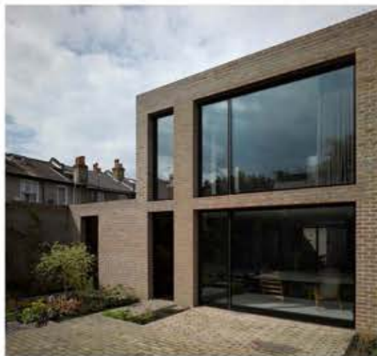
Precedent: Duggan Morris Architects - Kings Grove House. Grey/brown textured brick & header course, with large window recesses
