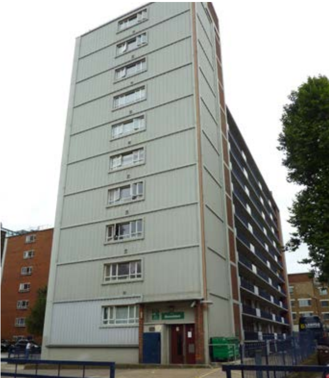
View of existing metal cladding to be replaced with brick and pre-cast concrete
