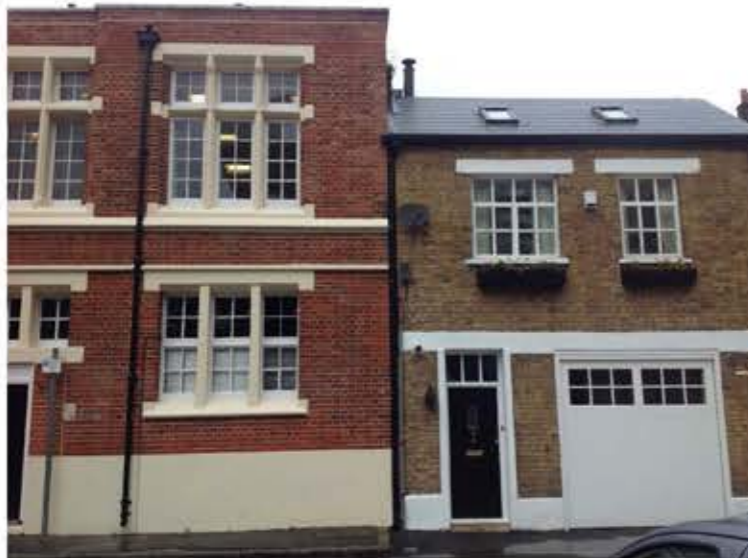
The addition of reconstituted stone cills & wall capping to the new houses will form a conversation with the existing mews houses at Barbon Close.
