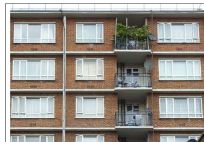
Horizontal concrete decks on Blemundsbury north elevation
