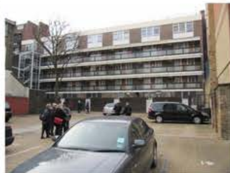
2- The existing space to the rear of Devonshire Court is dominated by car parking areas at present.
