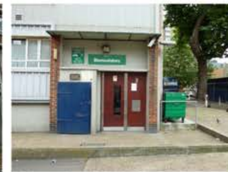
4- Entrance from Orde Hall Street adjacent to further external waste storage. Approach is blocked by kerb and level change.
