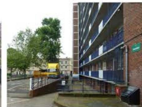
2- Existing ramped access and service area to the lower ground floor level of Blemundsbury to the north of the building.
