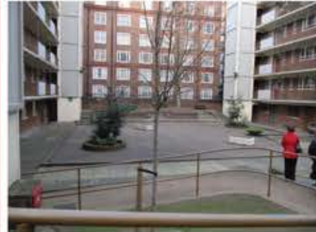
1- Existing courtyard viewed from south
