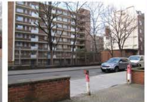
3- View of courtyard boundary from Boswell Street
