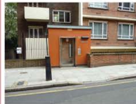
4- View of Falcon entrance from Old Gloucester Street with washrooms behind
