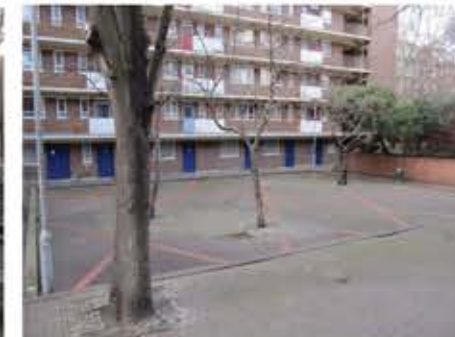
2- View of courtyard looking towards storage and TRA hall at lower ground.
