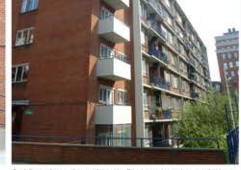
6- View from New North Street showing existing unused washroom balconies.
