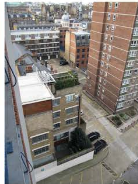
5- View of the spaces around Chancellor's Court and Devonshire Court as seen from the deck access of Blemundsburry, demonstrating the domination of hard standing and parking areas within these spaces.
