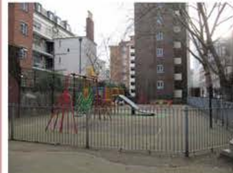
1- View looking south across play area showing north elevation of Falcon
