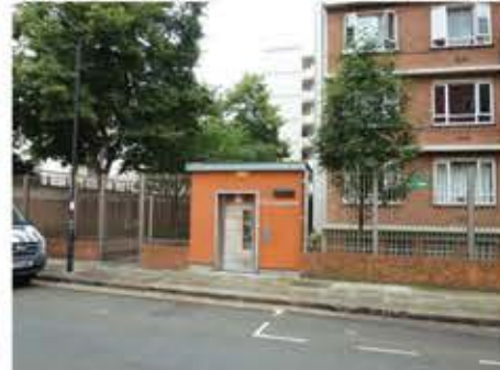
2- View showing entrance to Springwater from New North Street
