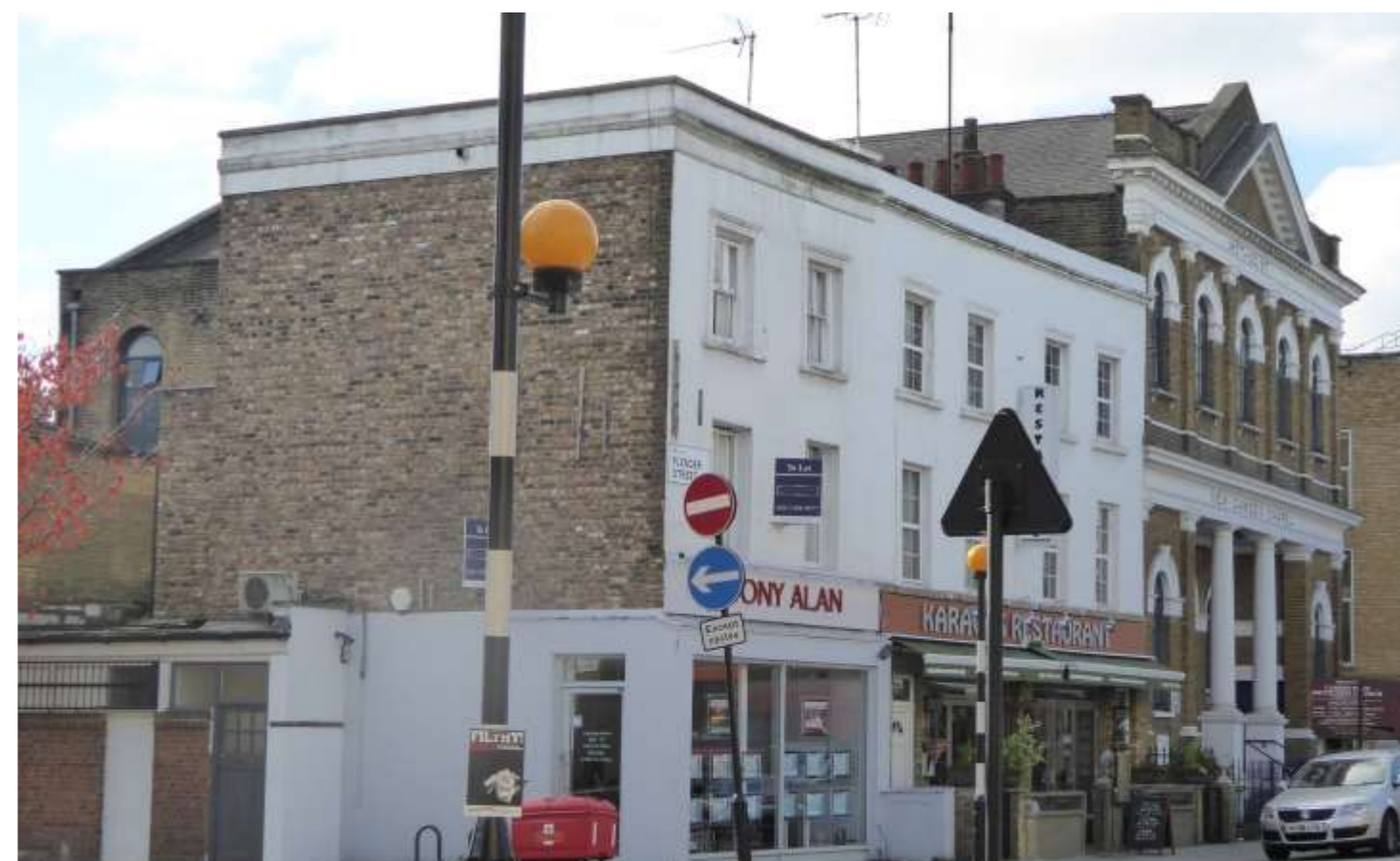
Plate 9: View from the east, showing the absence of a return to the facade.
