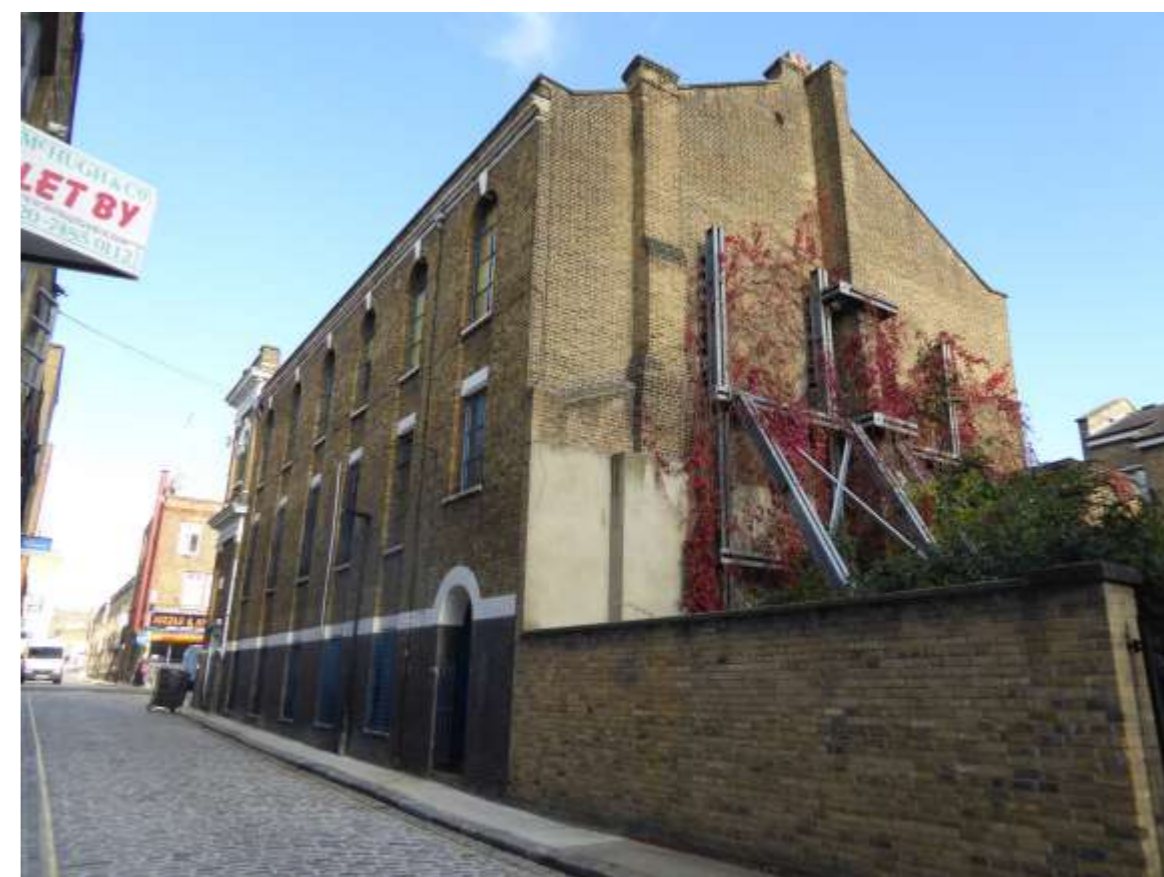
Plate 3: The south-west corner onto King's Terrace.
