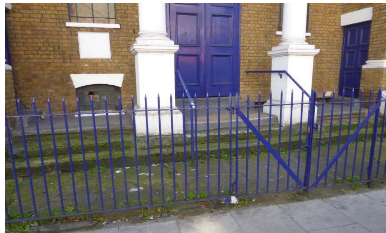
Plate 8: Detail of the steps at the main entrance.
