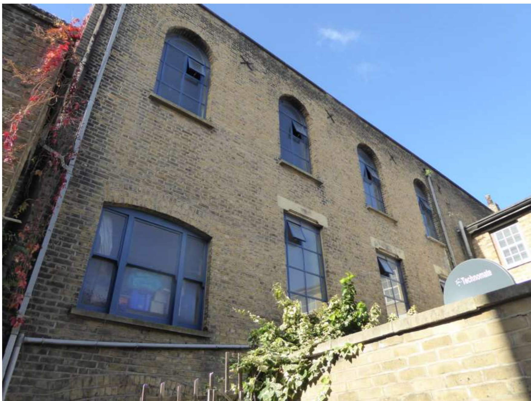
Plate 4: The upper part of the east elevation.
