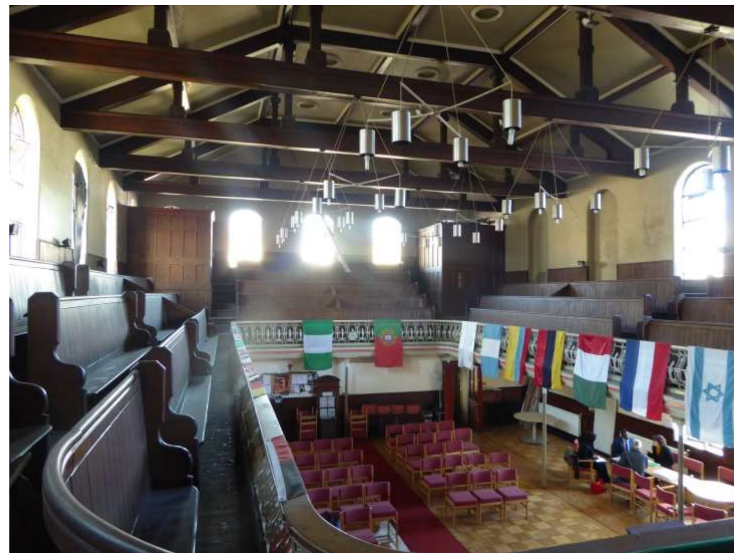
Plate 7: General view of the interior, looking north from the gallery.
