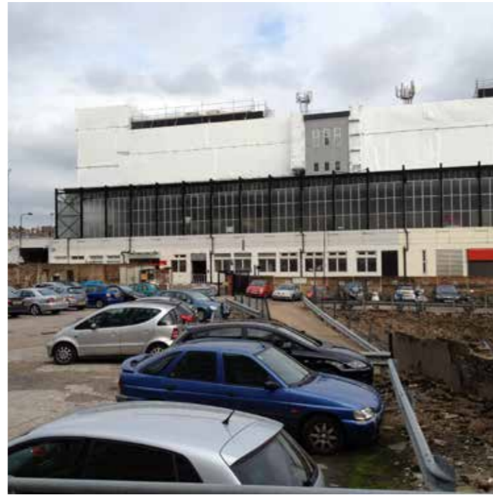
Phoenix Place looking north east
