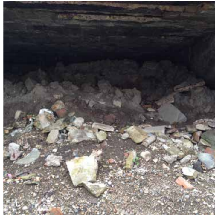
Vaults underlying Phoenix Place in the southern site corner
