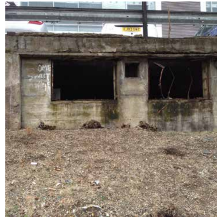
Vaults underlying southern corner of Phoenix Place
