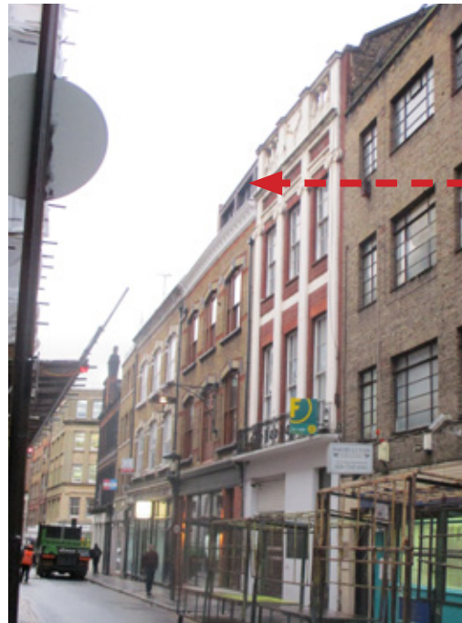
23 Hatton Wall - roof extension
