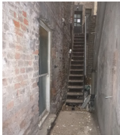
First floor window blocked up at the rear
