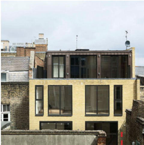
Metal clad roof extension at 23 Hatton Wall
