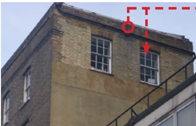
The facade is in a general state of disrepair. Remedial works are required to the windows, parapet and brickwork.
