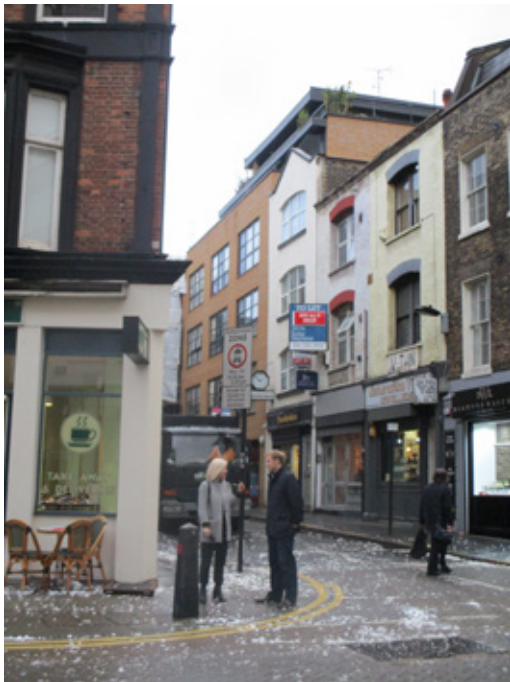
Hatton Wall - roof extension
