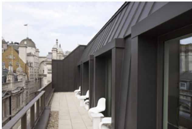
Eric Parry Architects, Piccadilly Black Zinc roof extension
