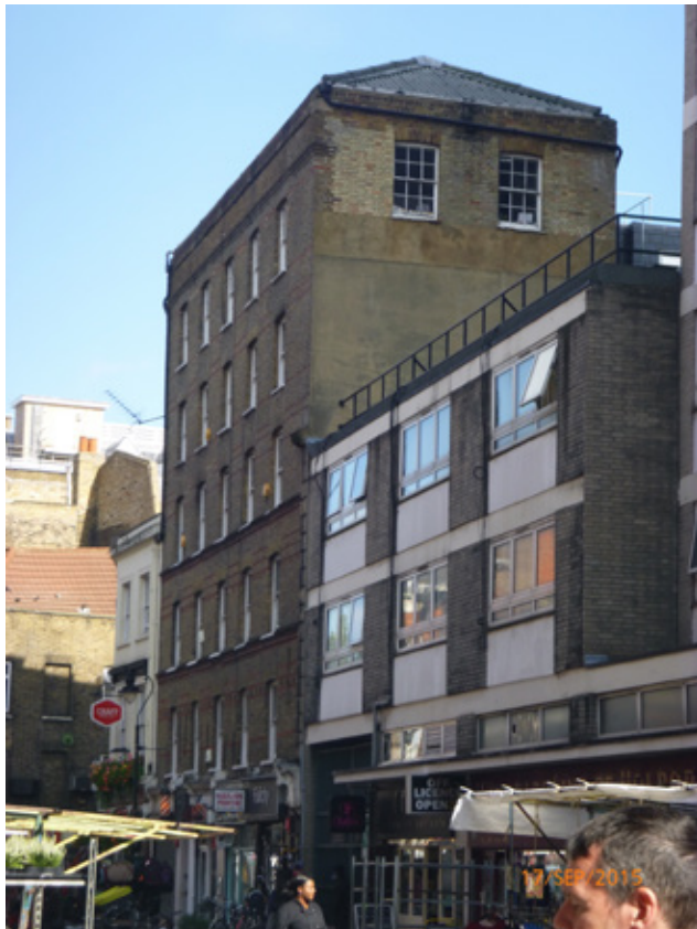
Existing building looking north along Leather Lane
