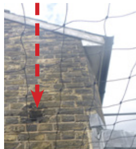
The facade is in a general state of disrepair. Remedial works are required to the windows, parapet and brickwork.
