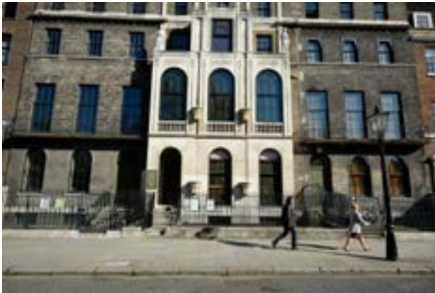
Figure 4: Existing signage to railings, May 2016
