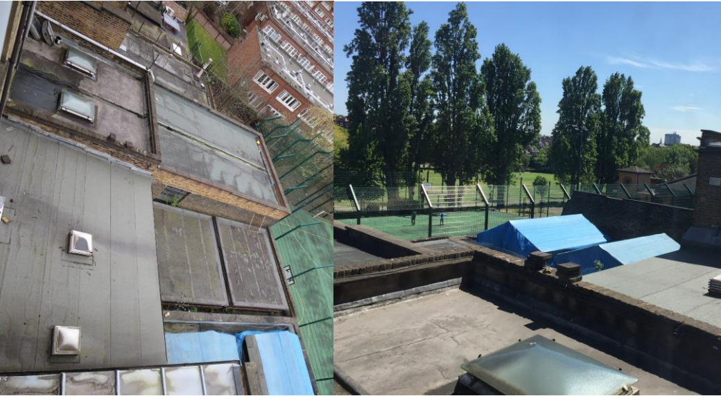
Photos showing the varied nature of the existing terrace
