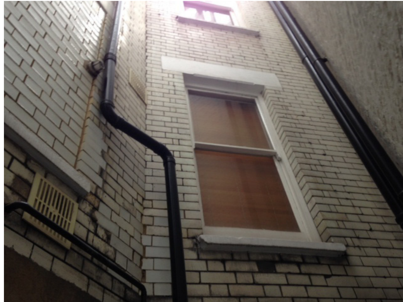
Photo existing Lightwell towards 12 Northington Street
