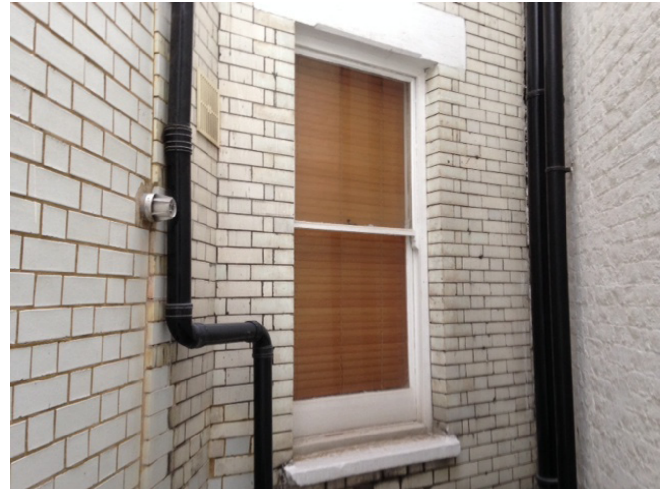
Photo existing Lightwell towards 12 Northington Street
