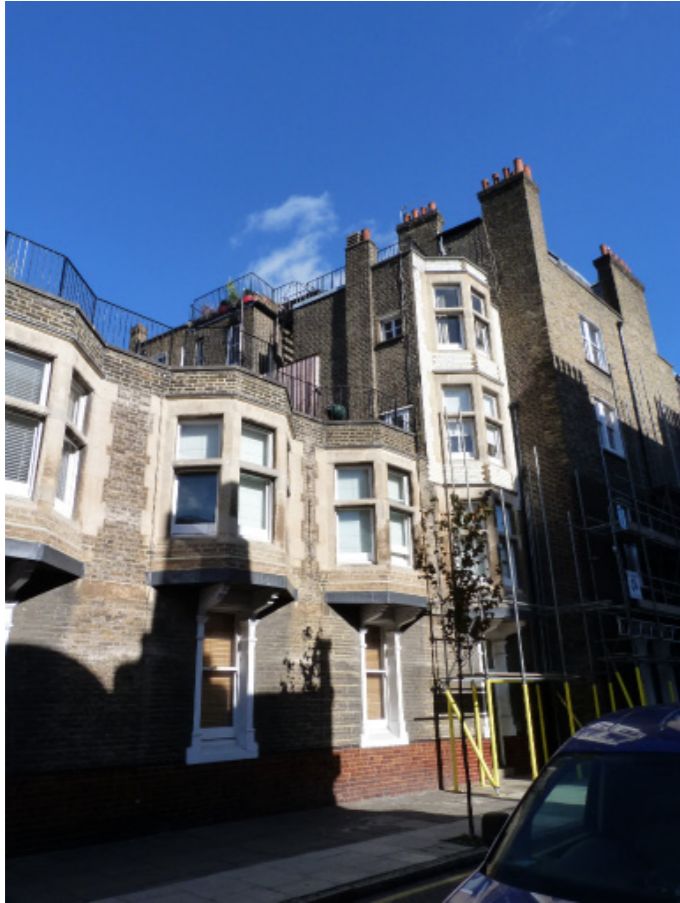
Front elevation 12 Northington Street
