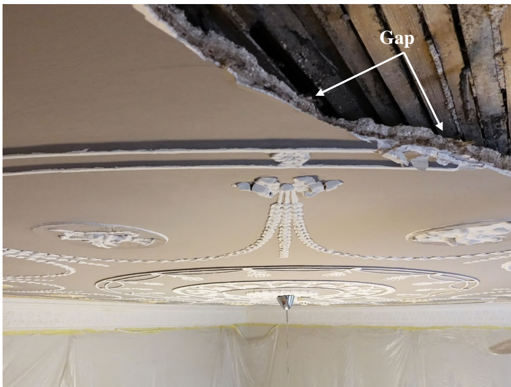
Fig. 08 Deflection of ceiling visible from NE view to SW
