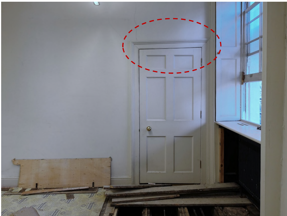
Fig. 18 Deflection of N-S partition and door distortion above on second floor
