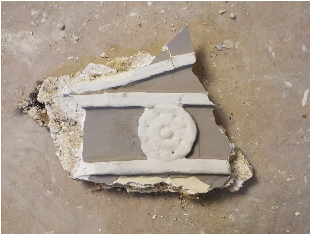
Fig. 11 Decorative cast plaster moulding applied to flatwork
