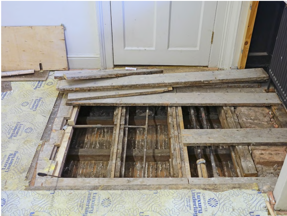
Fig. 27 Exposed ceiling back in east room NW corner 'B'
