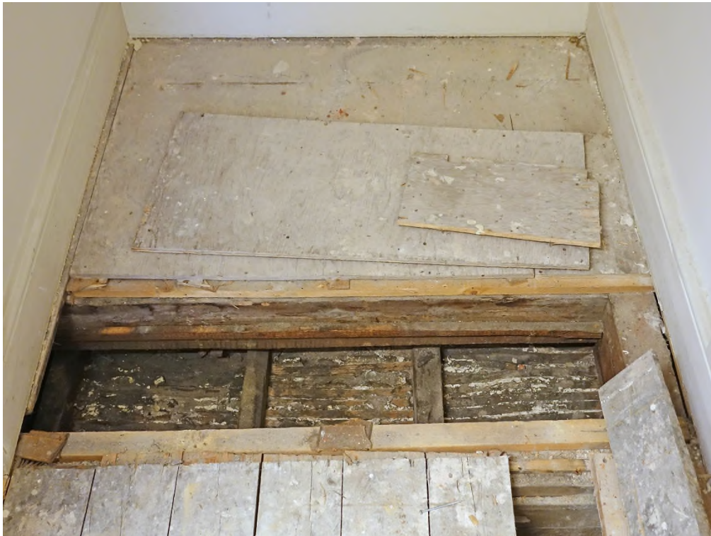
Fig. 31 Ceiling back exposed in SW corner cupboard of west room 'D'
