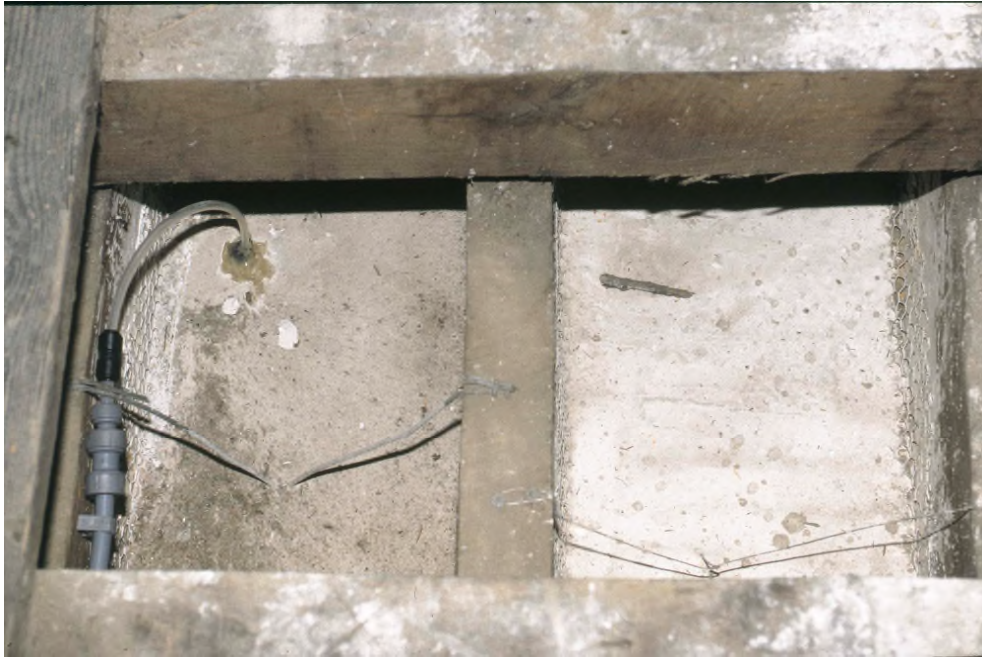
Plate A Illustrating inappropriate repair method applied to the back of an original ceiling (1605-08) at Knole House, Kent with poured plaster of Paris and chicken wire reinforcement together with galvanised wire ties passing through the ceiling face. The result is the wholesale obscuring of the structure beneath and creation of rigid inflexible blocks of plaster.
