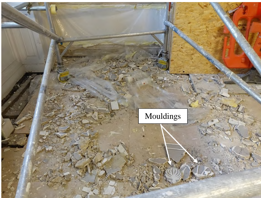
Fig. 04 Ceiling debris and mouldings on the floor
