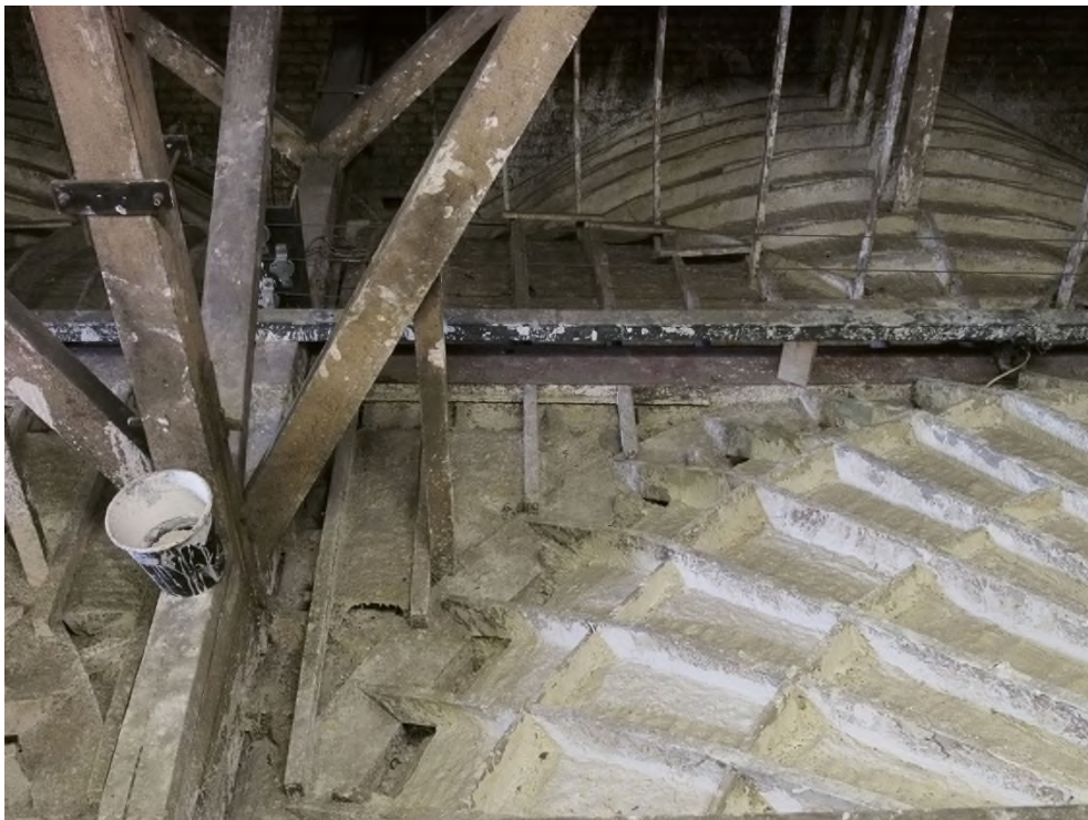
Plate B Illustrating inappropriate repair method applied to a nineteenth century lath and plaster ceiling with poured plaster of Paris and hessian reinforcement obscuring structure beneath, adding weight and reducing flexibility.
