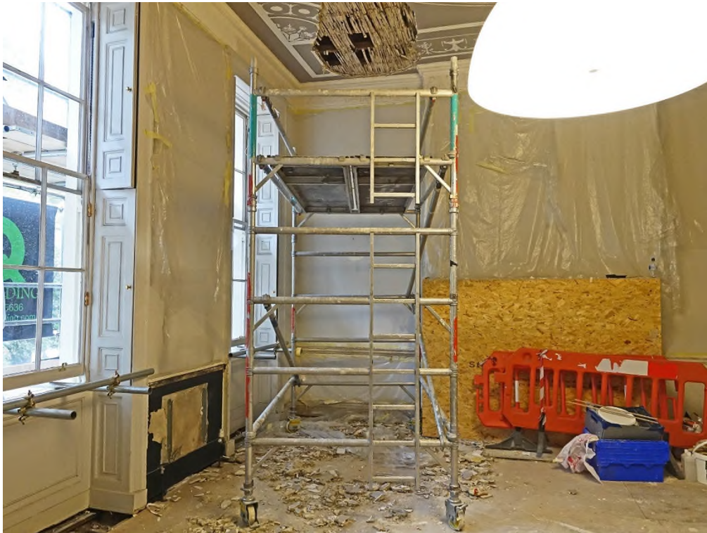
Fig. 03 Ceiling plaster loss in NE corner
