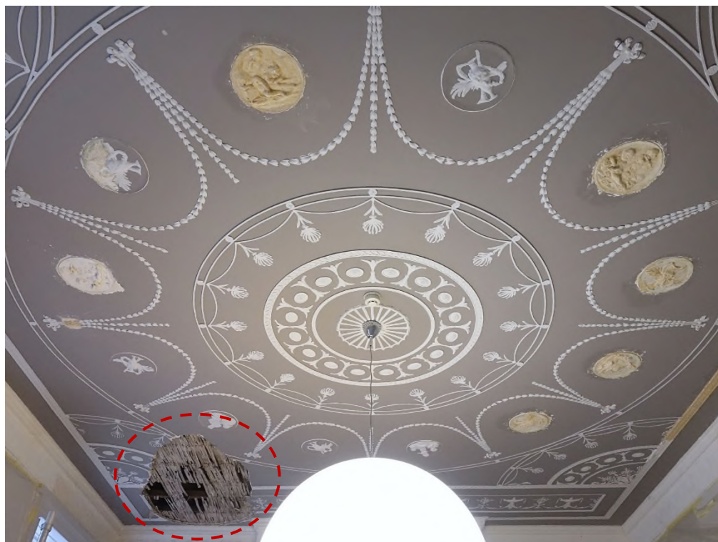
Fig 02 First floor front ceiling view east with plaster loss 15/10/16
