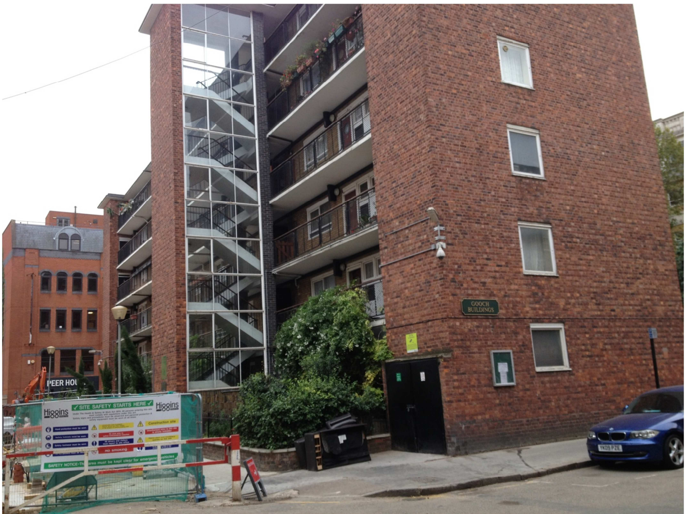
Plate 1: East elevation of the Gooch Building block illustrating the enclosed communal staircase
