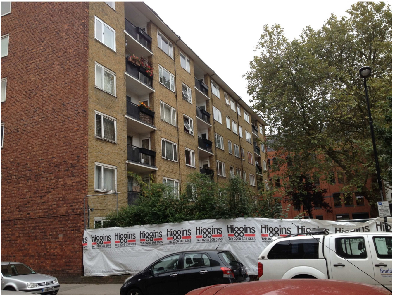
Plate 2: West Elevation of the Gooch Buildings illustrating the timber casement windows
