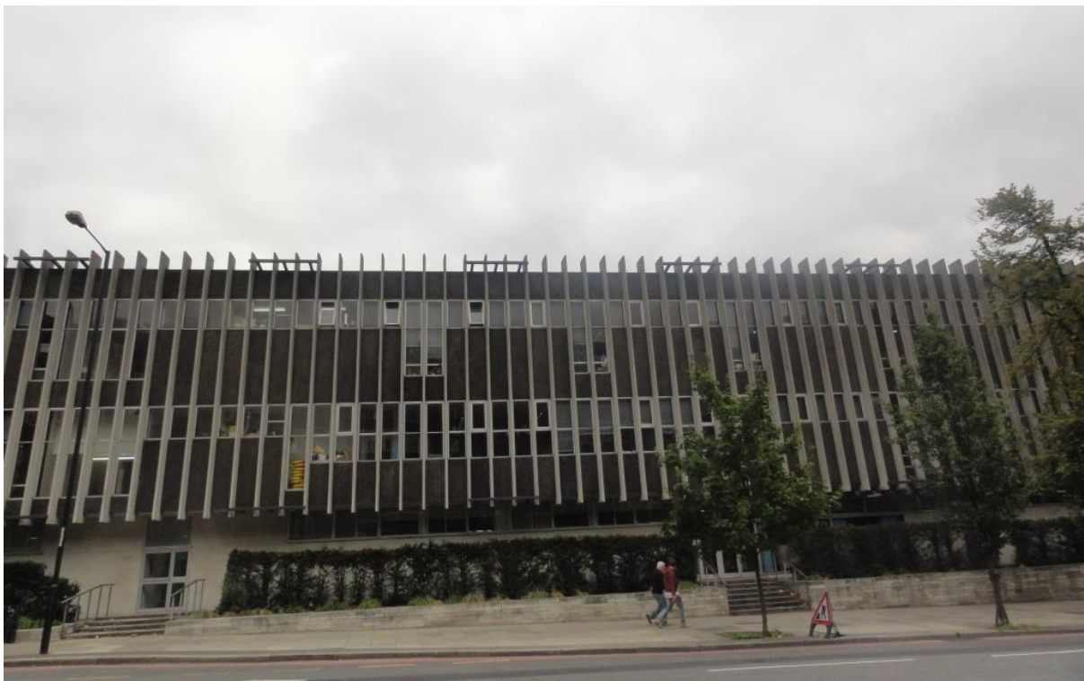
Figure 8. Finchley Road view – the panels cannot be seen.
