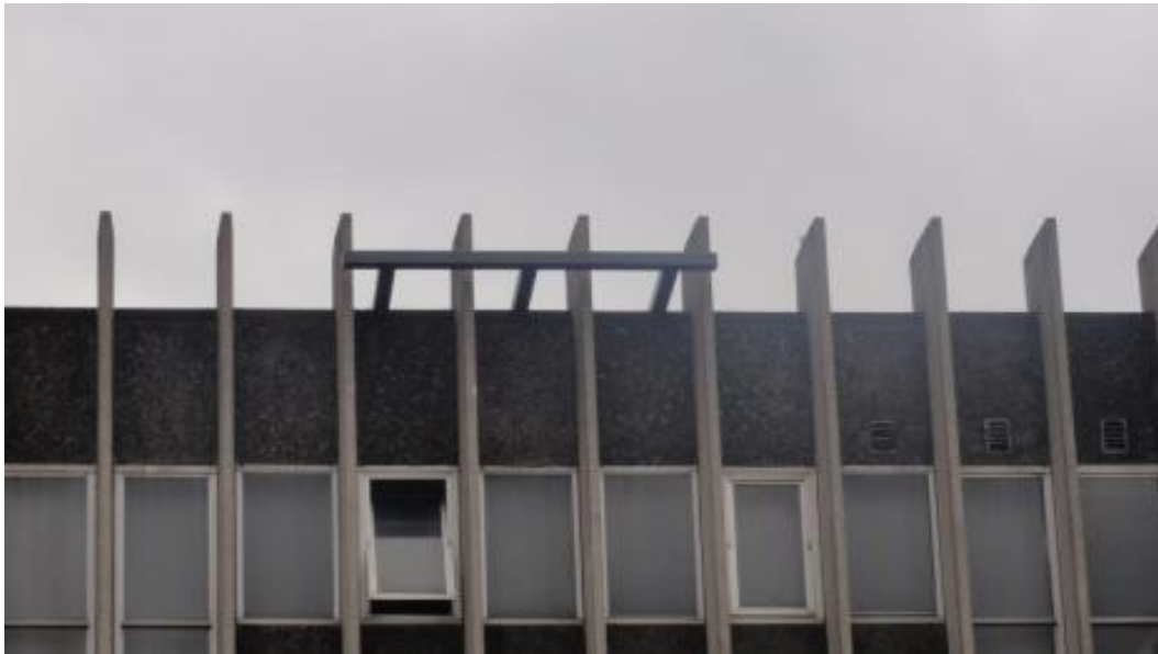
Figure 9. Finchley Road view – the panels cannot be seen.
