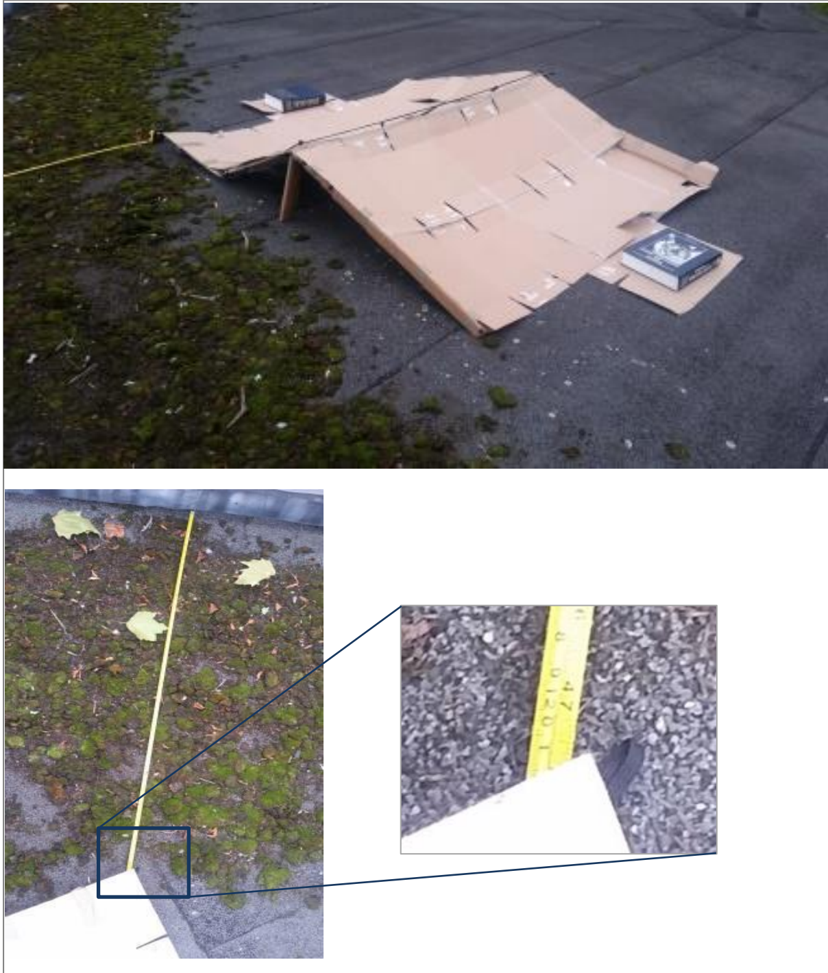
Figure 1. Set of mock cardboard solar PV panels set 1.2m away from the edge of the roof.
