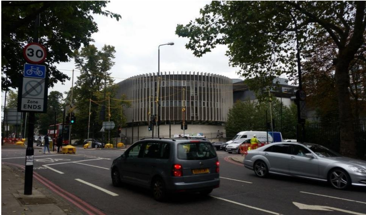
Figure 13. Adelaide Road view – the panels cannot be seen.
