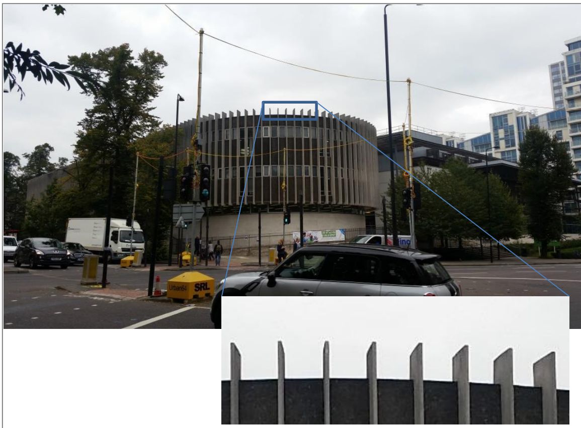
Figure 12. Adelaide Road view – the panels cannot be seen.
