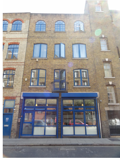
Photo B: Front elevation to previous extension
