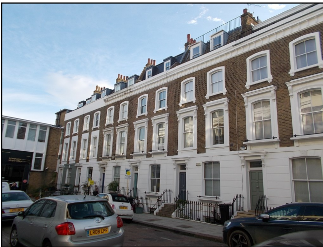
Street scene showing other mansard roof extensions adjacent to the site
