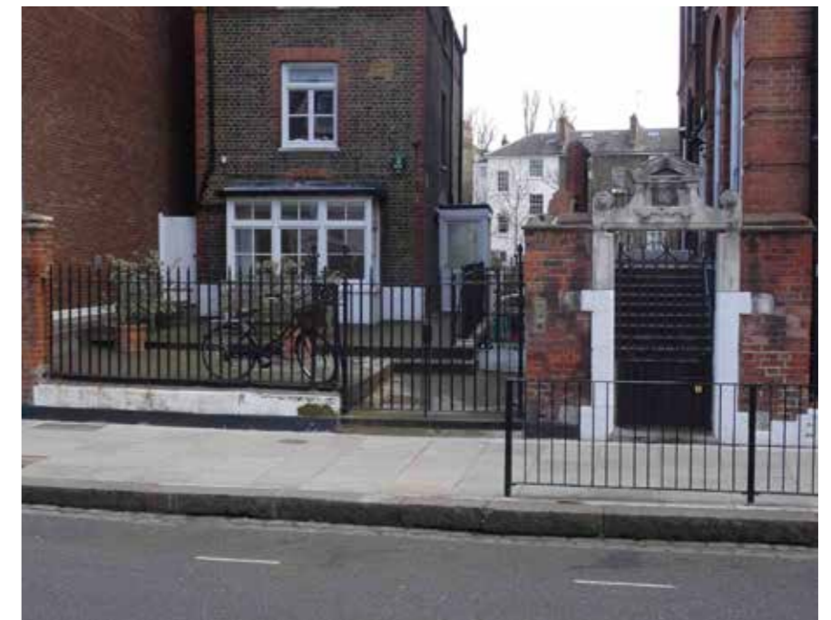
View from the street of the Caretaker's House and main building. The gates installed in 2011 are to be fixed shut. The revised entrance for the two year-old unit is to be through the Boys gate to the right.
