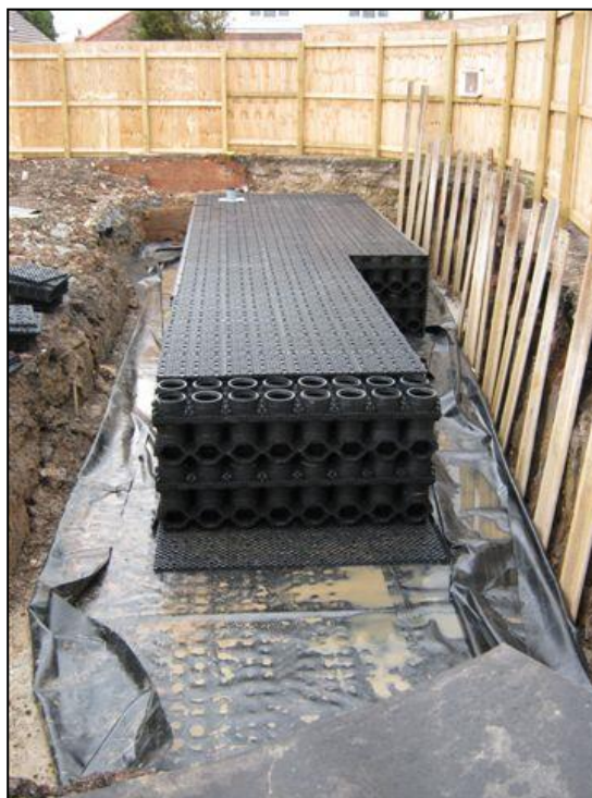
Figure 3.1: A typical cellular attenuation tank
