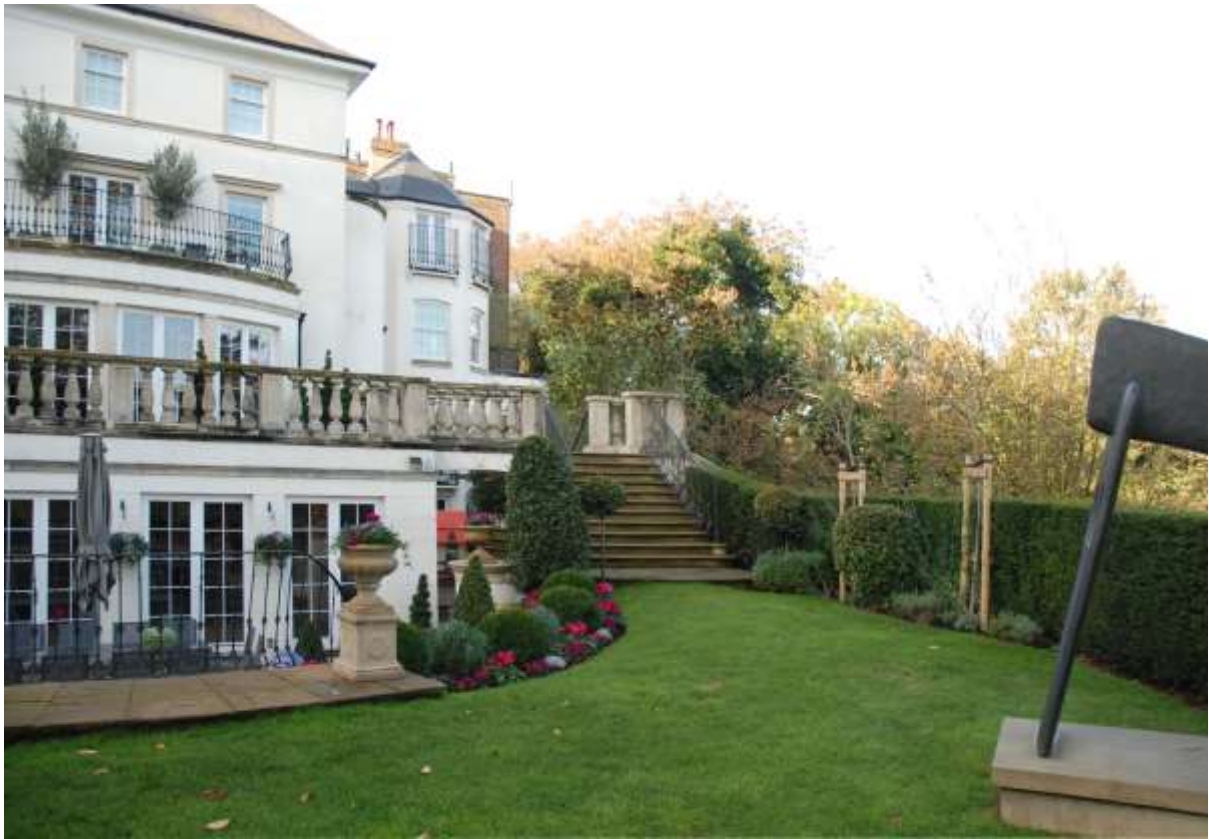
Fig.33: Shot 2. Exterior of Whitestone House. Facing NW
