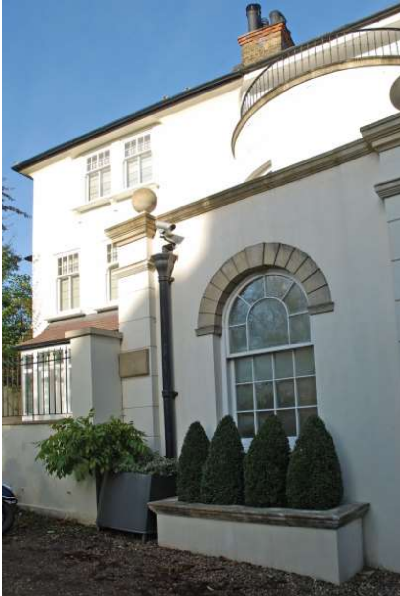
Fig.44: Shot 13. The south face of Whitestone House. Facing SW.
