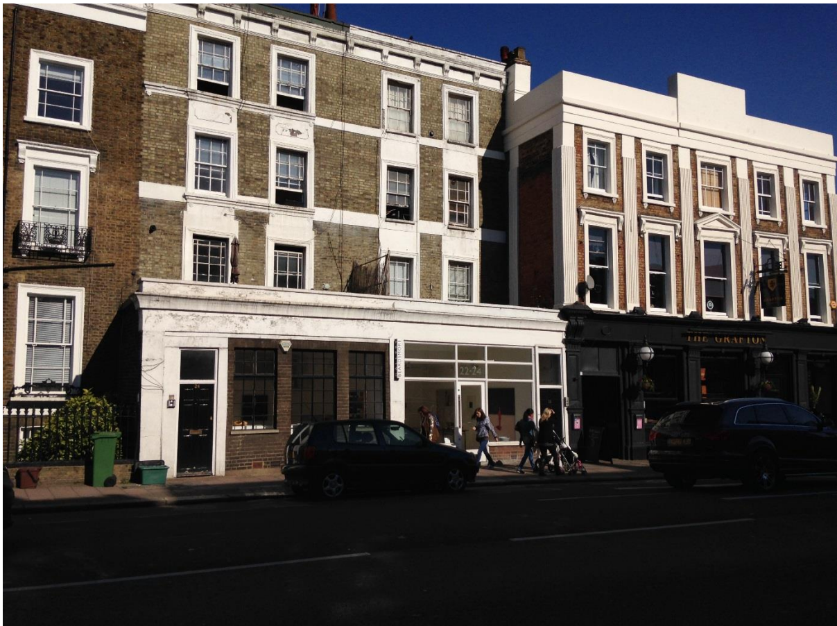
View of the building from Prince of Wales Road
