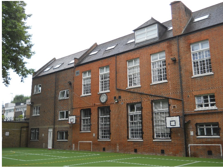
Photo 4: East side of main building.
