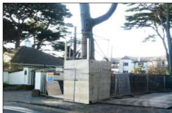
Fencing image 6: Board secured to scaffold framework adds another layer of protection for vulnerable trunks and branches
