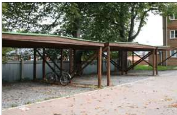
New structure image 1: These carports are formed by wooden posts above a three dimensional cellular no-dig and load-spreading surface of permeable crushed stone.
