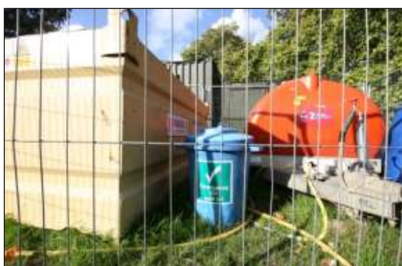
Pollution image 1: Where fuel or other chemicals are stored on site, it is now standard practice to have emergency spillage kits available to restrict the environmental impact of accidents.
