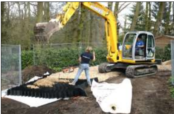
Ground protection image 5: Cellular products are a very effective means of providing ground protection where heavy vehicle use is expected. Here, it is being used to temporarily widen an existing road, to be removed once the construction is finished.
