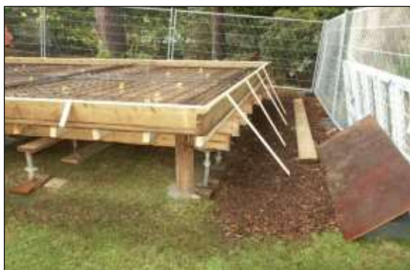
New structure image 3: Small diameter piles (less than 150mm) are an effective means of supporting structures in RPAs with minimal disturbance.
