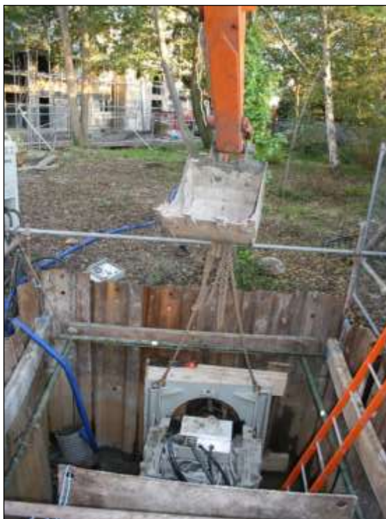
Services image 1: If possible, thrust boring is the preferred option for installing service routes through the RPAs of important trees, but there has to be space at the start and finish to dig substantial working pits.
