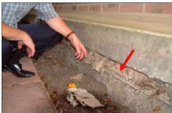
New structure image 9: Where a slab is cast on site, a biodegradable void-former (red arrow) temporarily supports the weight of the liquid concrete until it sets. The void-former can then be wetted and washed away to leave a void or left to degrade naturally, both of which allow movement of air beneath the slab.
