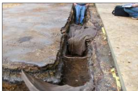
Excavation image 4: Exposed roots must be protected from light, drying out and extremes of temperature by covering with hessian sacking and boards until they can be covered back with soil.
