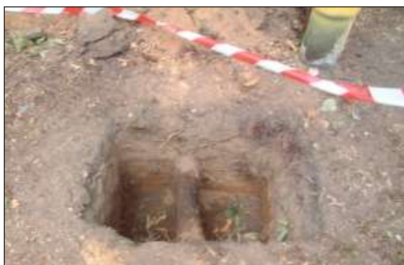
New structure image 5: Where piles are proposed close to trunks, it is essential to excavate 50–75cm deep to see if there are any significant roots in the way, with provision to move the pile location if roots are found (note the pile was finally installed to avoid this root).
