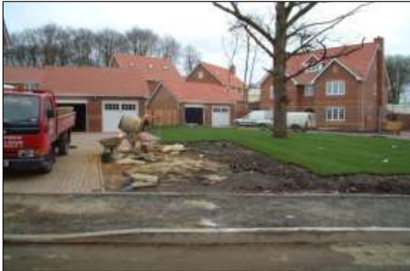
Landscaping image 1: The RPA of this tree was not effectively protected during construction and excessive compaction of the soil meant it died soon after this turf covered up the damage.
