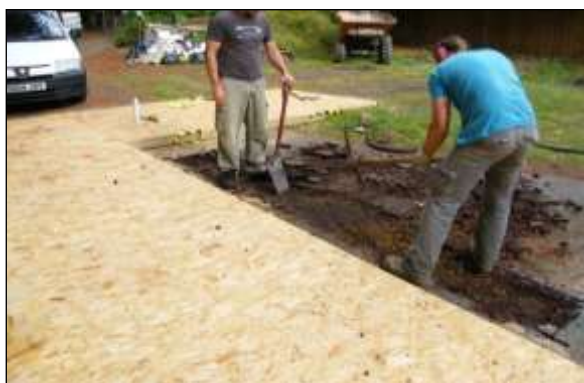
Excavation image 1: Careful hand-digging using conventional tools is acceptable for exposing roots in RPAs.
