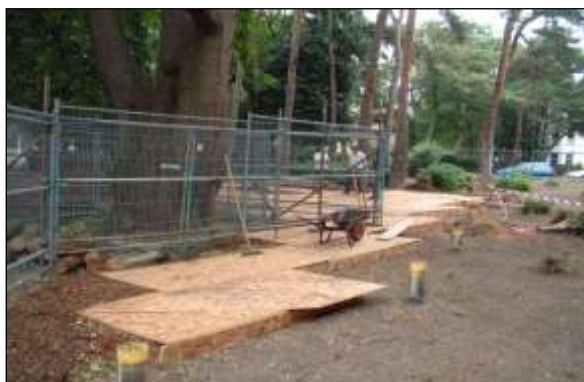
New structure image 7: Once the piles have been installed (yellow tops), the ground protection to support the piling rig is removed ready to fix the void-former onto the bare soil, in advance of pouring the building slab.
