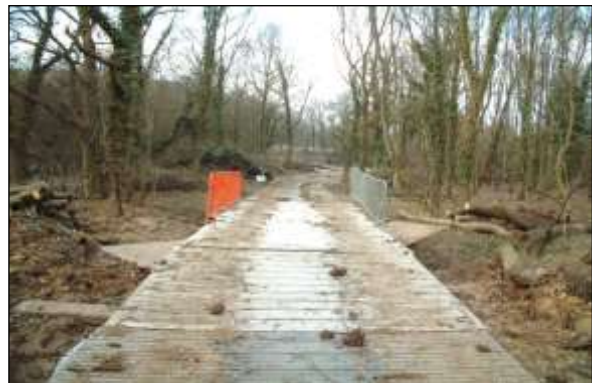
Ground protection image 6: Custom designed sectional tracks can be joined to support very heavy traffic use through sensitive areas.
