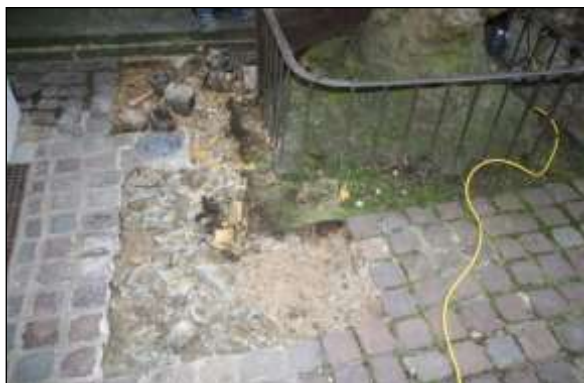
Hard surfacing/structure removal image 3: Careful lifting of cemented-in sets round this tree allowed them to be re-laid on a permeable sand base, improving the water input into the soil around the trunk.
