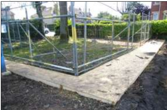
Ground protection image 3: Plywood fixed to a wood frame is another effective method of protecting soil from pedestrian compaction.
