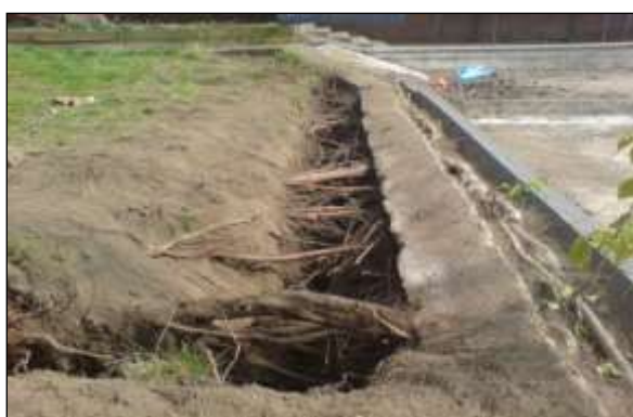
Excavation image 3: Air spades are particularly useful where roots are very dense.
