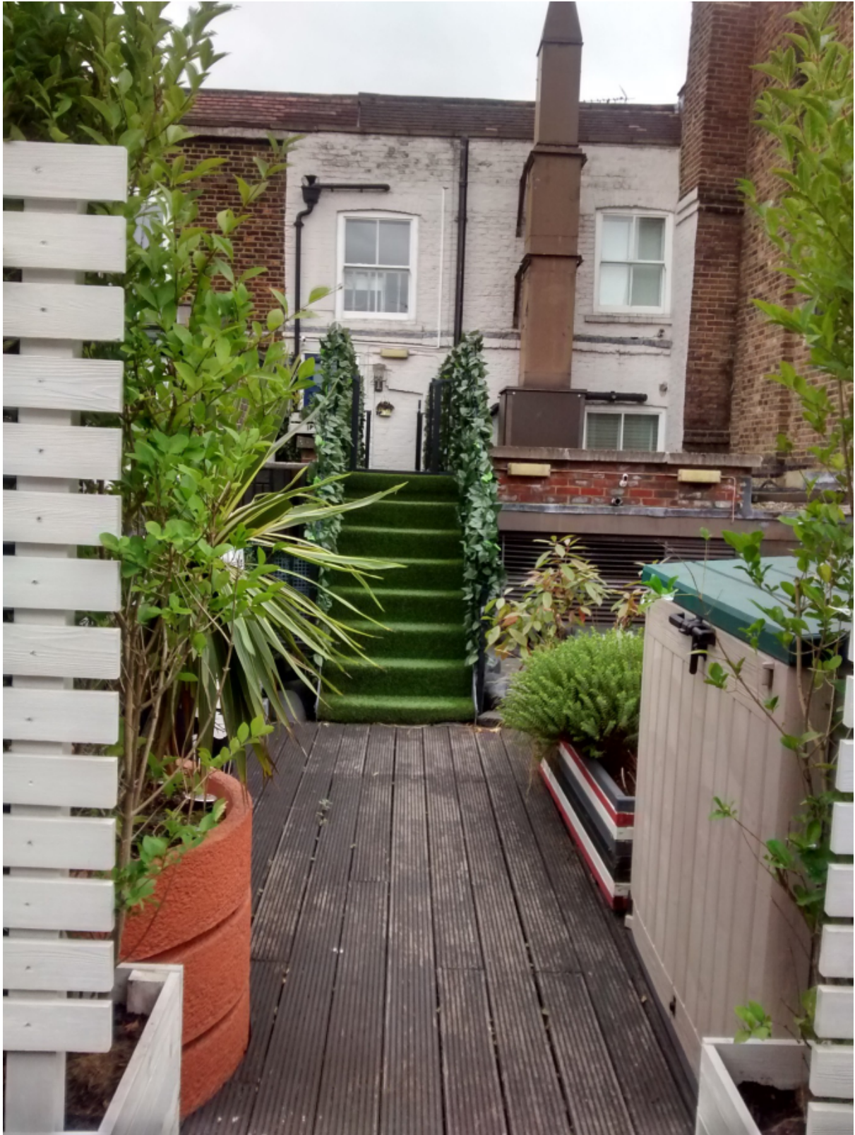
4. Looking south west towards the rear elevation of 46 Hampstead High Street, with views of the existing roof
