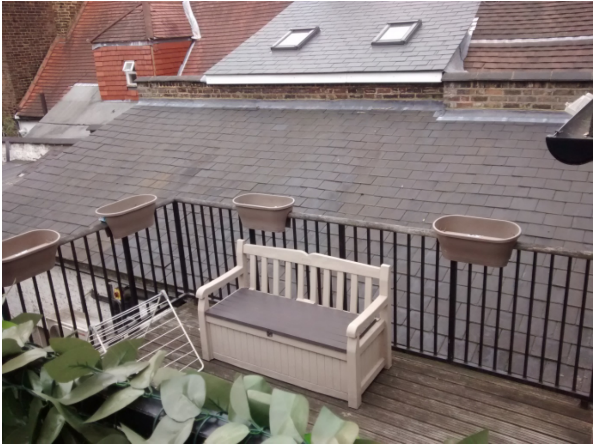
6. Looking south east towards the terrace at no. 45 Hampstead High Street
