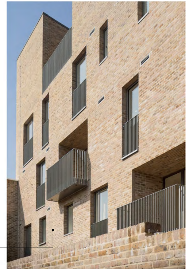
London Stock brickwork
