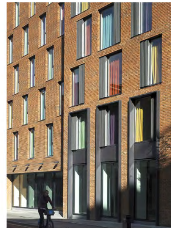
Example use of glass and metal louvres by Lifschutz Davidson Sandilands
