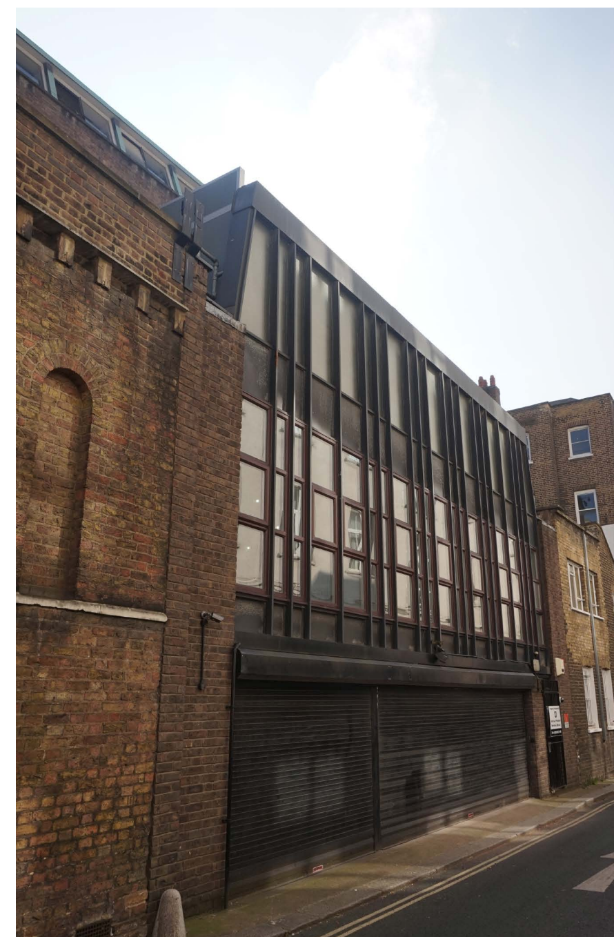
Curtain Walling at application site
