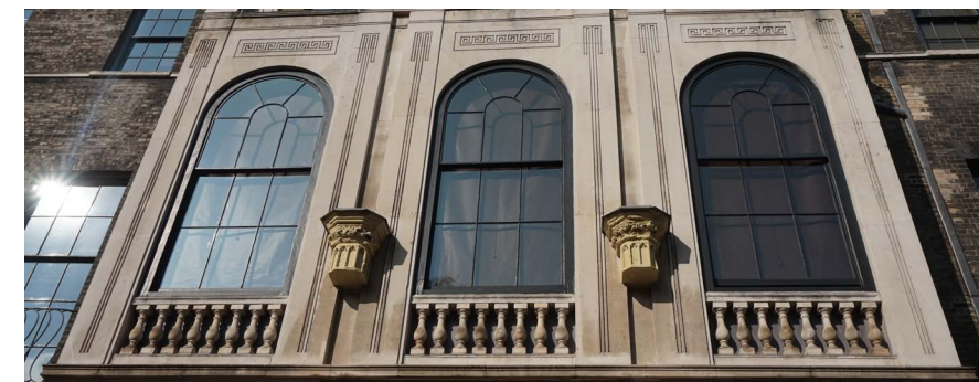
Portland stone loggia with ornate blind balustrade
