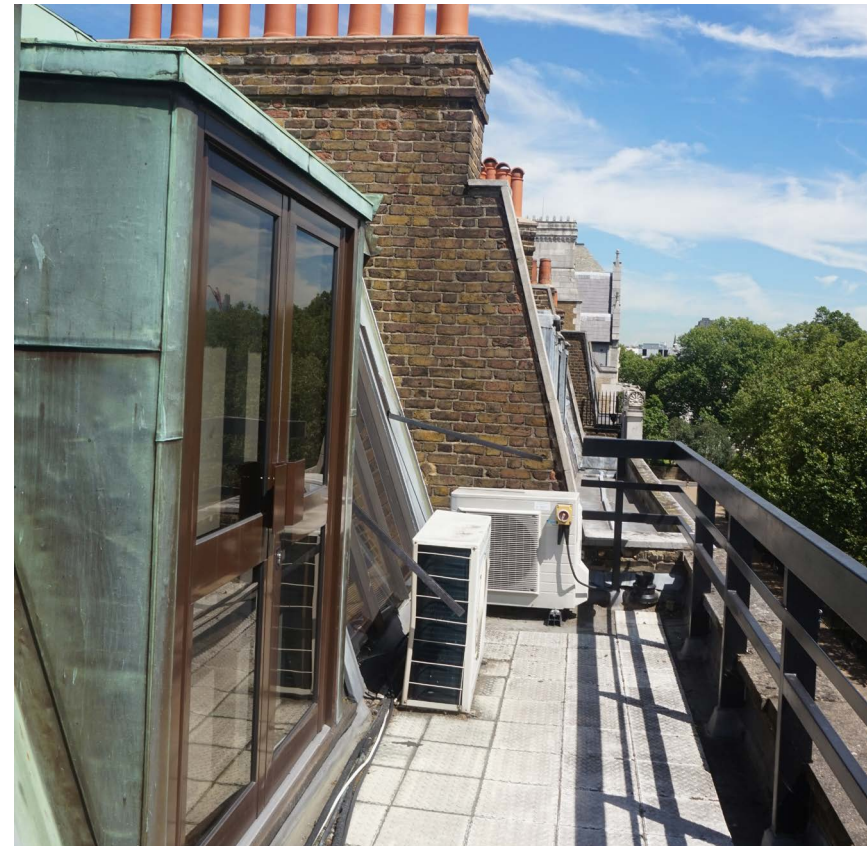
Plant clutter to 5F terrace and metal balustrade
