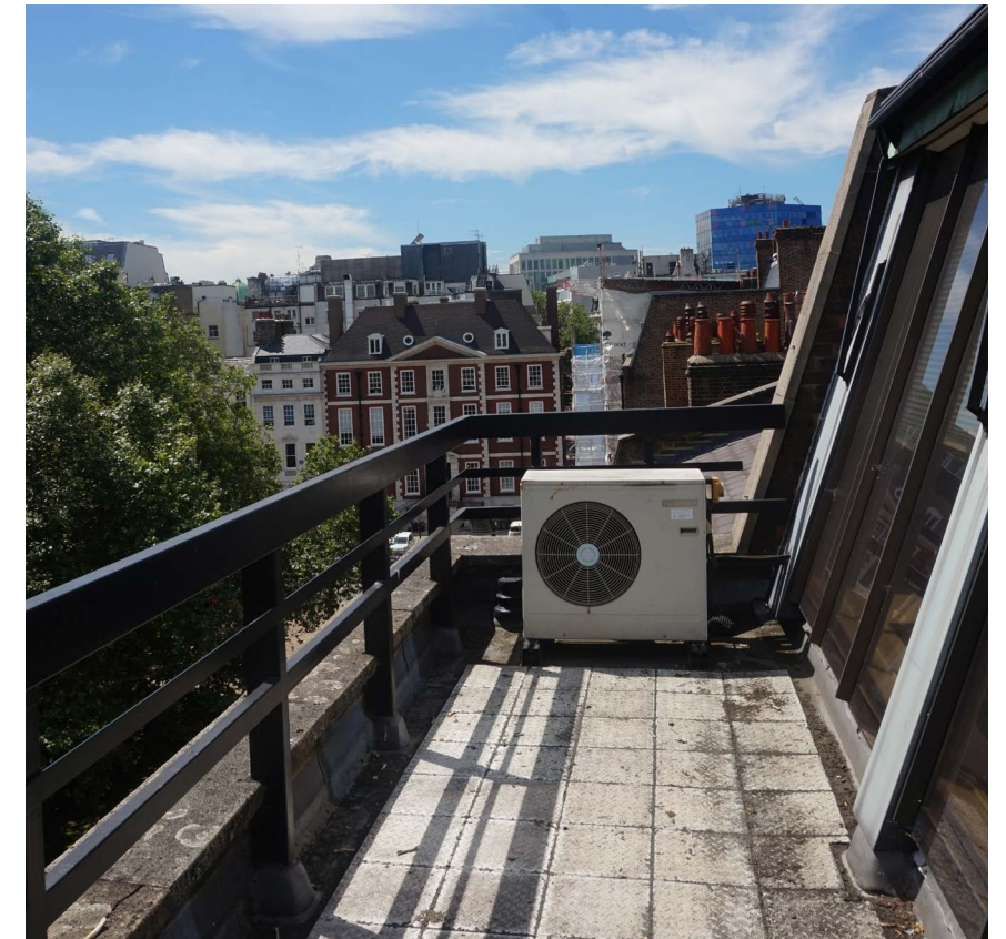
Plant clutter to 5F terrace and metal balustrade
