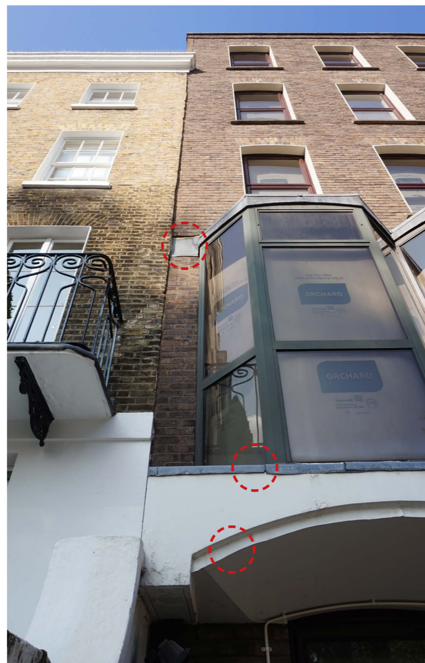
Front Facade - Junction to No.9 showing retrofitted lead details
