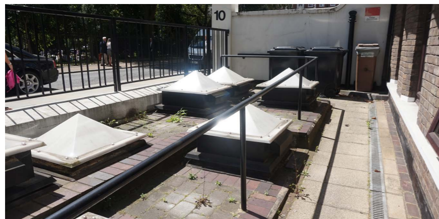
Front "Streetscape" - PVC pyramid roof-lights, ramps and bins
