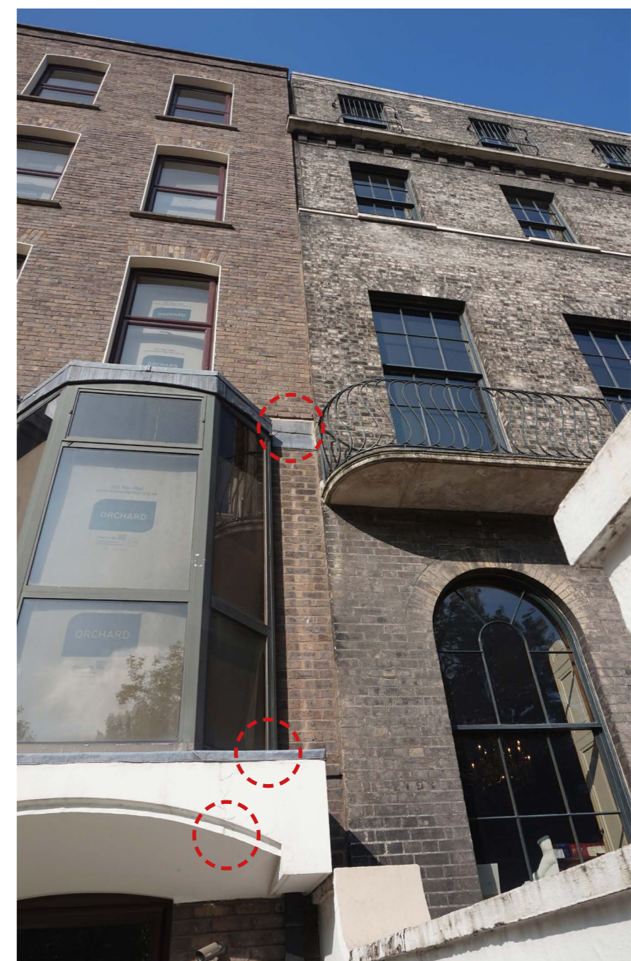
Front facade - Junction to No.12-14 showing retrofitted lead details
