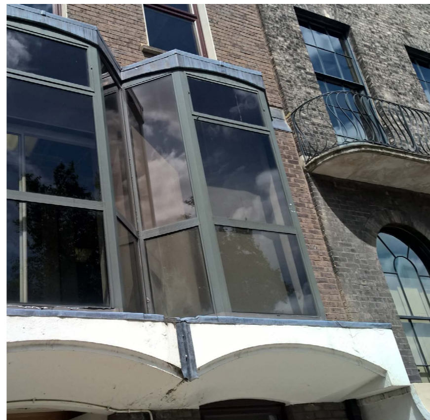
1F Bay Windows with concrete canopy and added lead details
