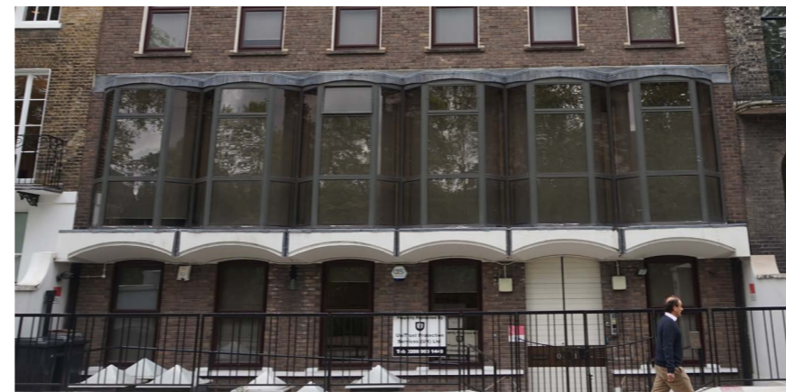
1F Bay Windows with secondary glazing
