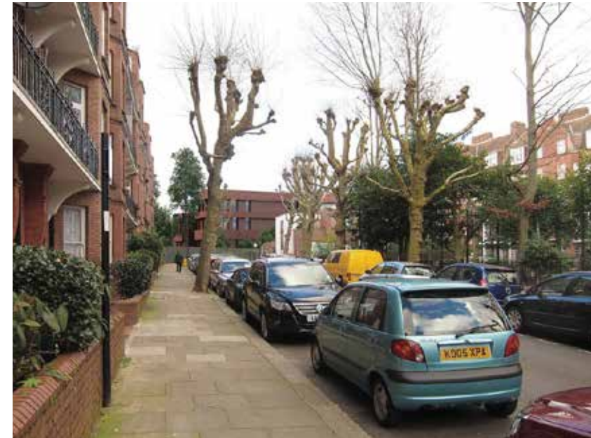
Proposed view from Lissenden Gardens towards Parliament Hill School showing new teaching block behind The House
